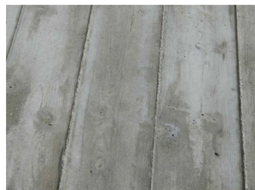
CLEAR-SEALED BOARD-FORM CONCRETE OR PORCELAIN TILE VENEER AT COLUMNS
