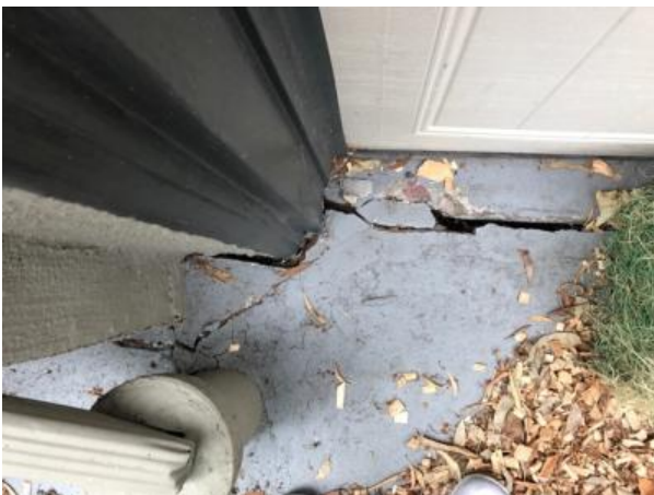
Photo 3: Crack in front of the garage that extends across the entire front of the garage
