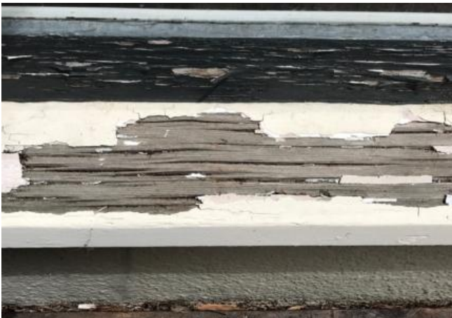
Photo 12: Sill damage on center picture window
