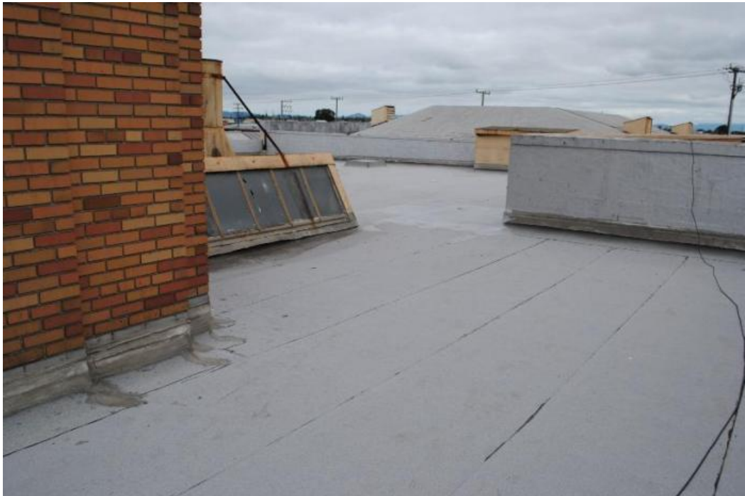
Counter-flashing work at tower connection to roof.
