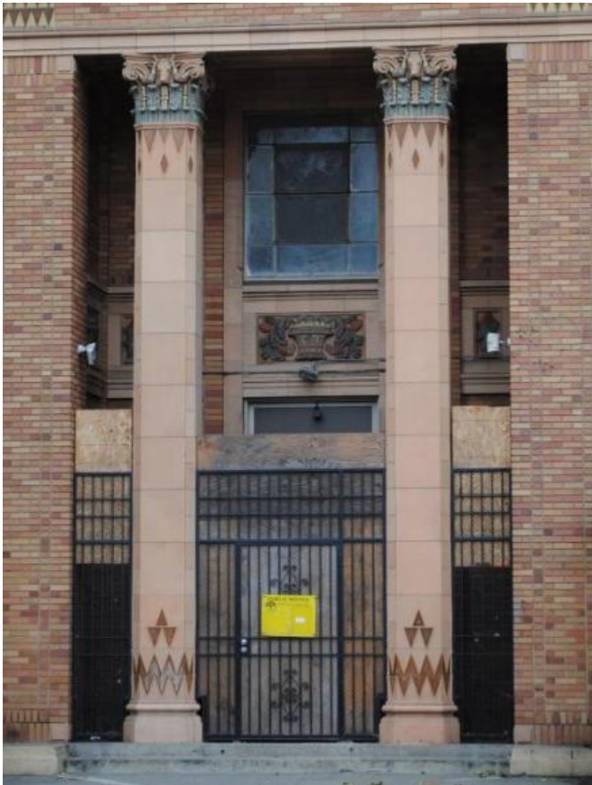
Replacement of iron grill at main entry with more compatible design.
