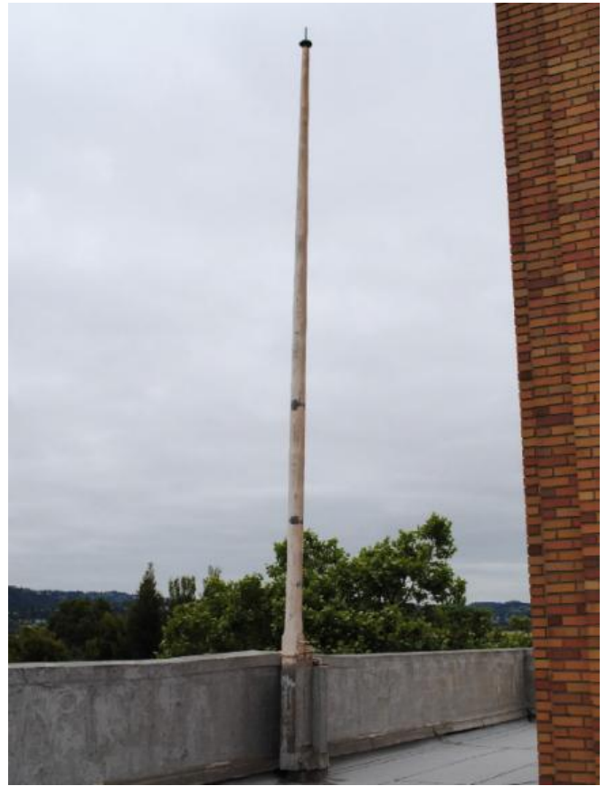
Restoration of flagpole, including preparation for priming and repainting, and new hardware.
