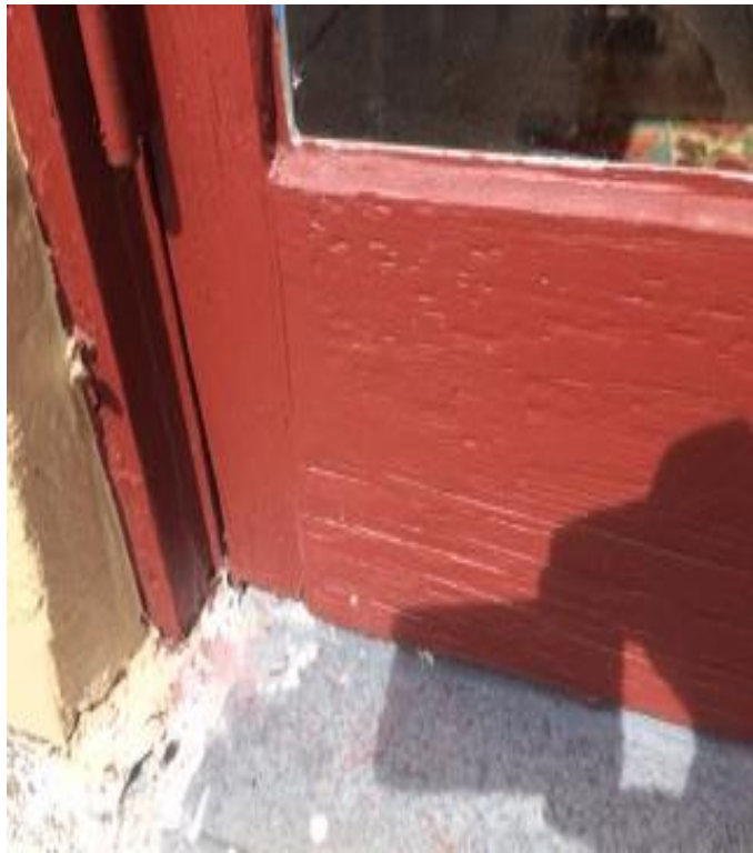
Wood rot on doors and windows
