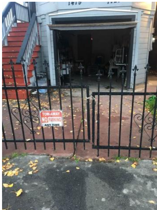
PHOTO H – Work Items 8-9 - Front fence in need of replacement; tied together with rope because latch does not work
