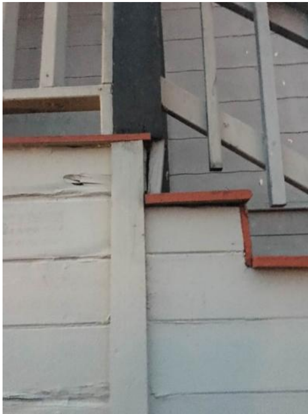
PHOTO G – Work Items 8-9 - Front staircase in need of repair/replacement
