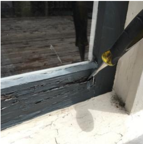
Photo 14: Right window of picture window, frame completely rotted
