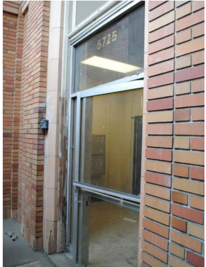
Replace primary entry door and window assembly on primary (north- east) facade with a compatible assembly. View from exterior.
