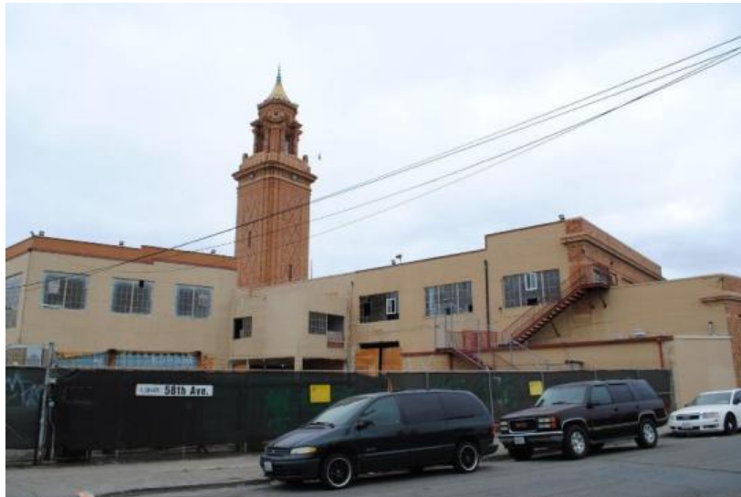
Rear (southwest) facade of the primary wing, looking north
