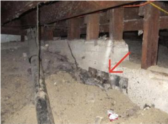
Photo 4: Crack covered by steel strap and spalling
