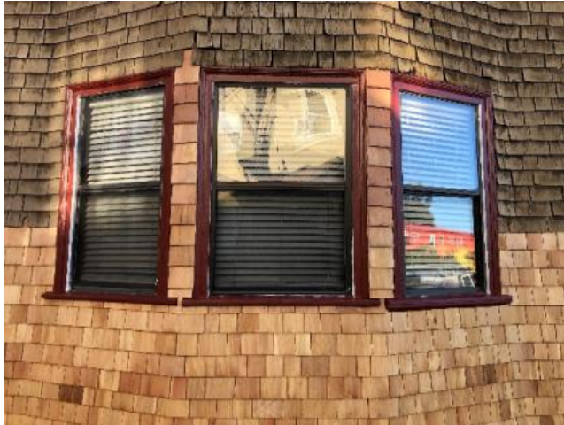
Lower (528) side bay windows – recent partial replacement of shingles and painting of sills performed by owners
