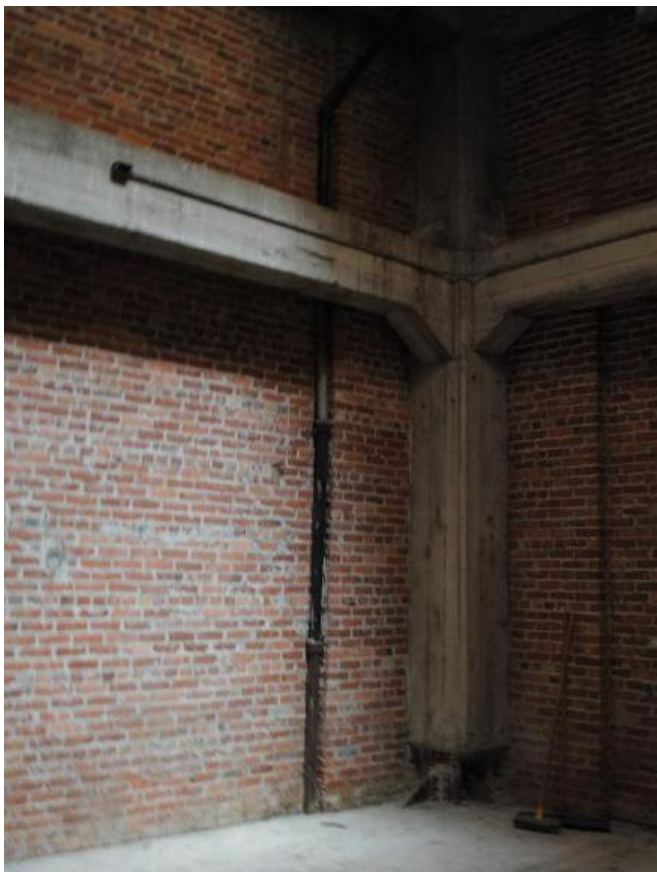
Seismic bracing of tower: interior walls shear improvements.
