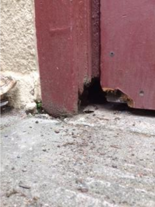
Garage Door Rot and Fungus
