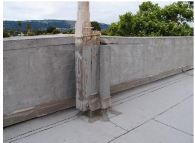
Restoration of flagpole, including counter-flashing at roof.
