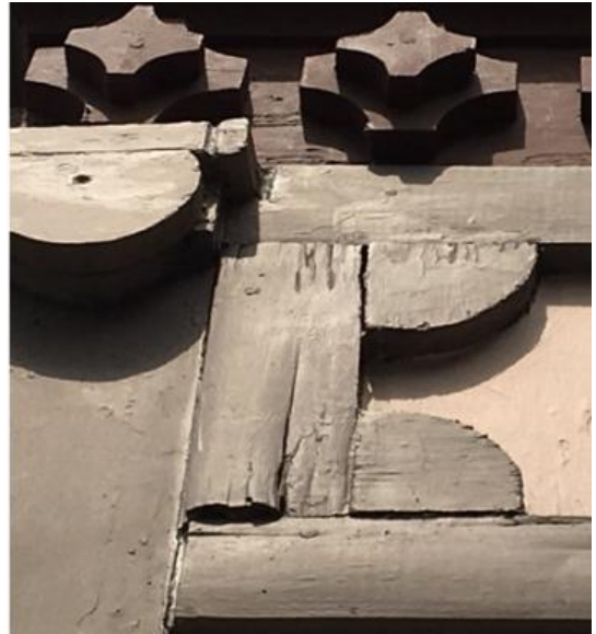
Faux-Victorian appliques mixed with original surfaces, windows, brackets
