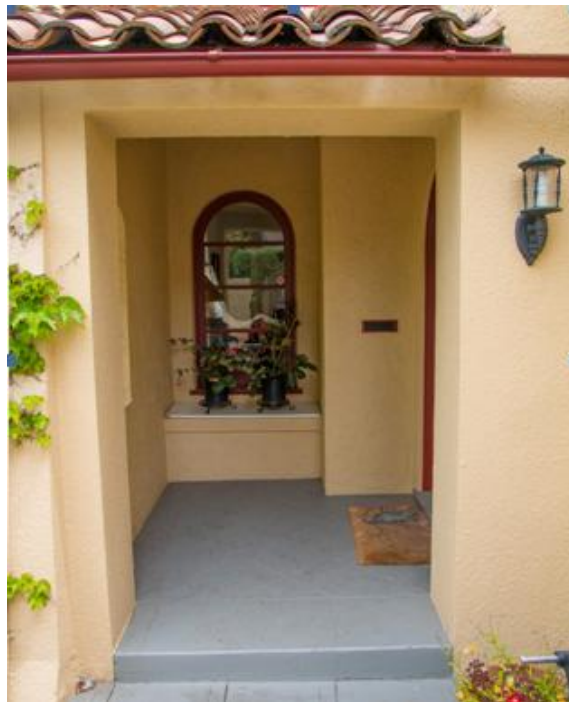
Recessed entry; tile roof
