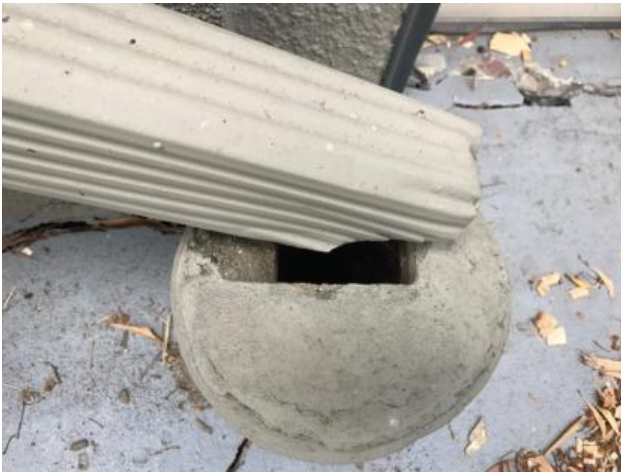
Photo 9: Clay drainage appears to be original
