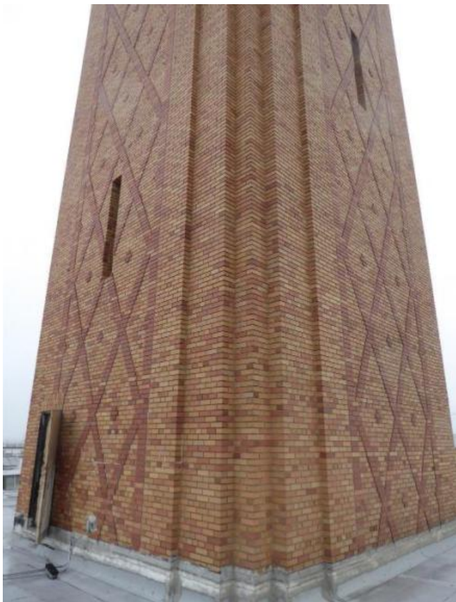
Seismic bracing of tower: foundation work. View of tower base at roof.
