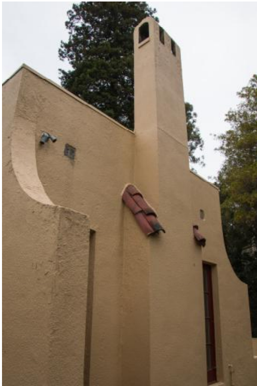
Chimney in danger of collapse
