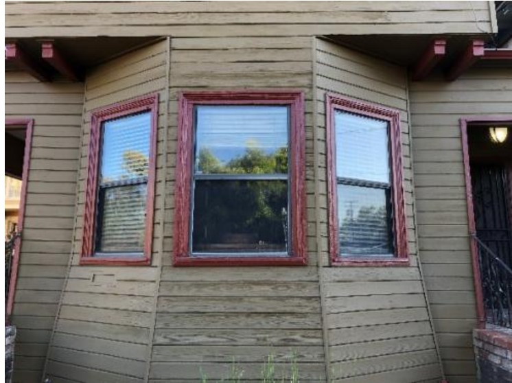
Shingles and trim to be restored
