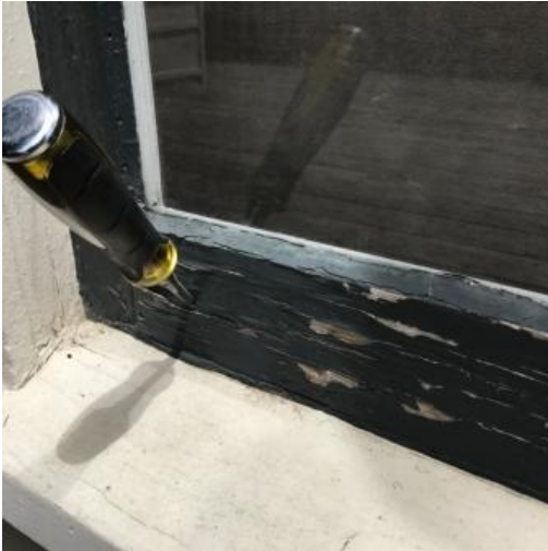
Photo 13: Left window of picture window, frame completely rotted
