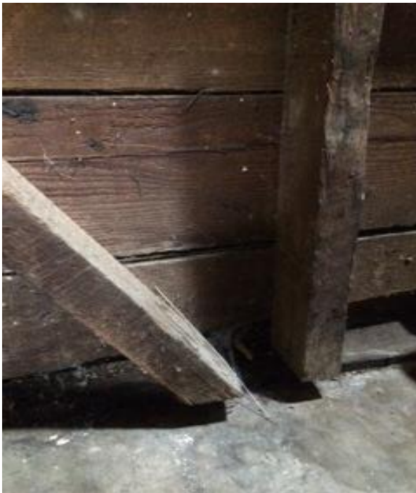
Garage separating from foundation
