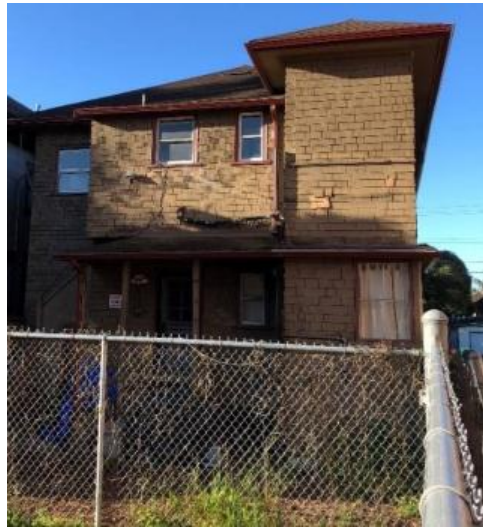
View from rear (behind neighbor's fence)
