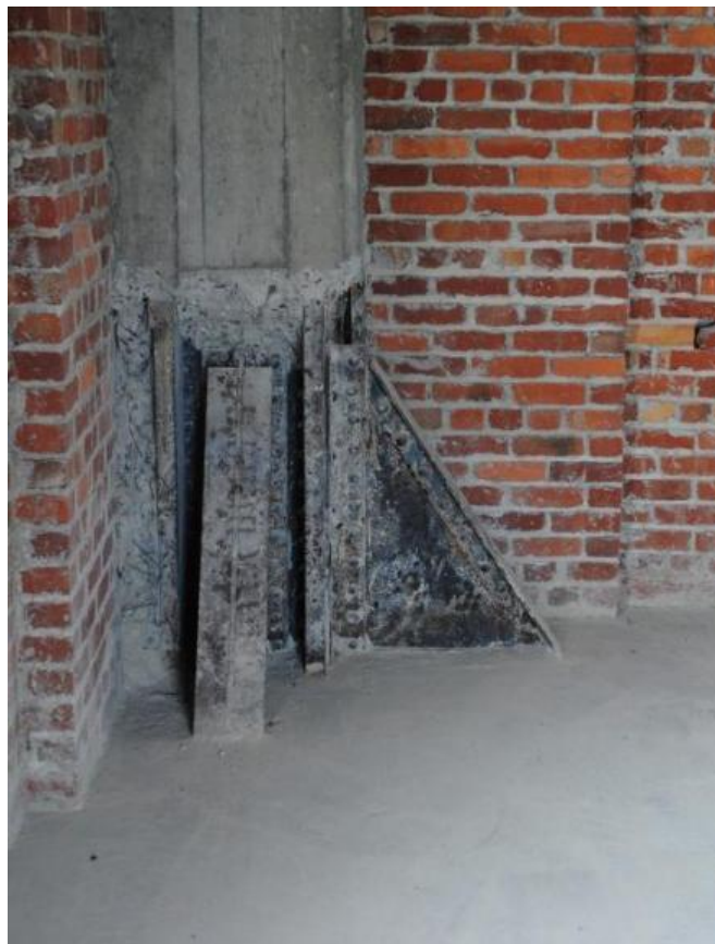
Seismic bracing of tower: foundation work. View of concrete and steel structure at interior of the tower.
