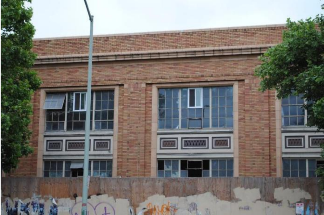
Removal of non-original window elements, and replacement with compatible inserts.
