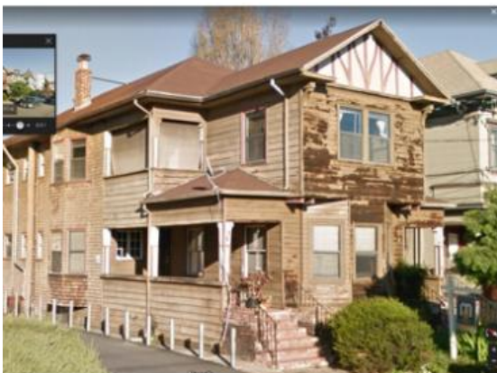
View of 528 28 th St from southwest corner (Dec 2016 – Google Street View)
