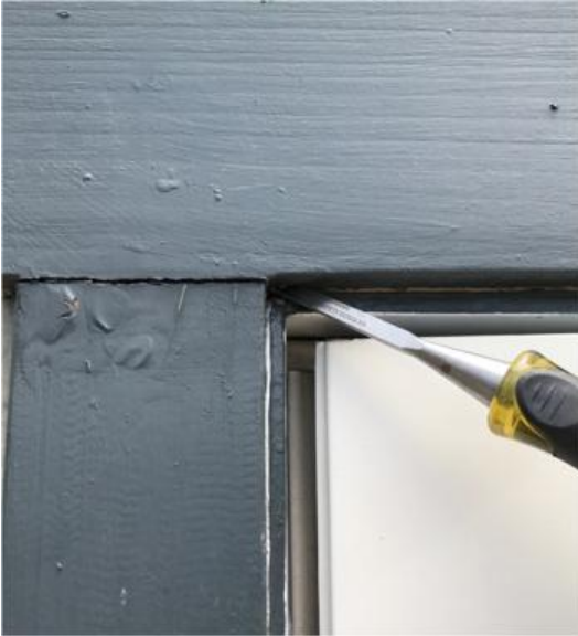
Photo 18: Frame rot on French door
