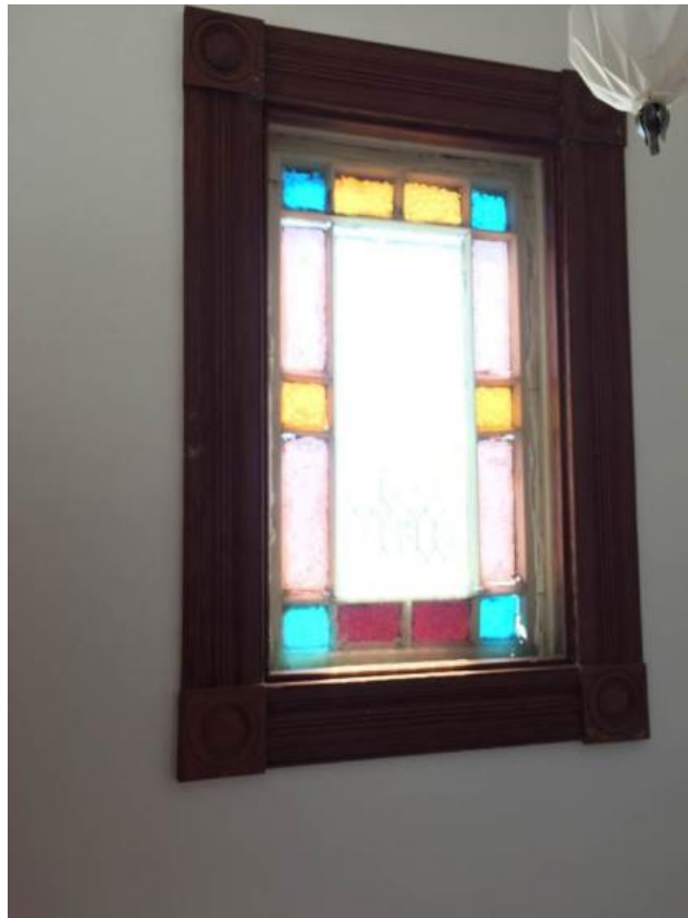
PHOTO I – Work Item 10 - Stained glass window in entryway with significant damage. Currently covered with plexiglass on both sides as temporary preservation mechanism.
