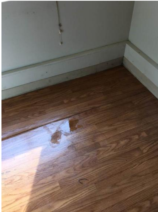
PHOTO F – WORK ITEMS 6-7 – Water intrusion in Lower unit
