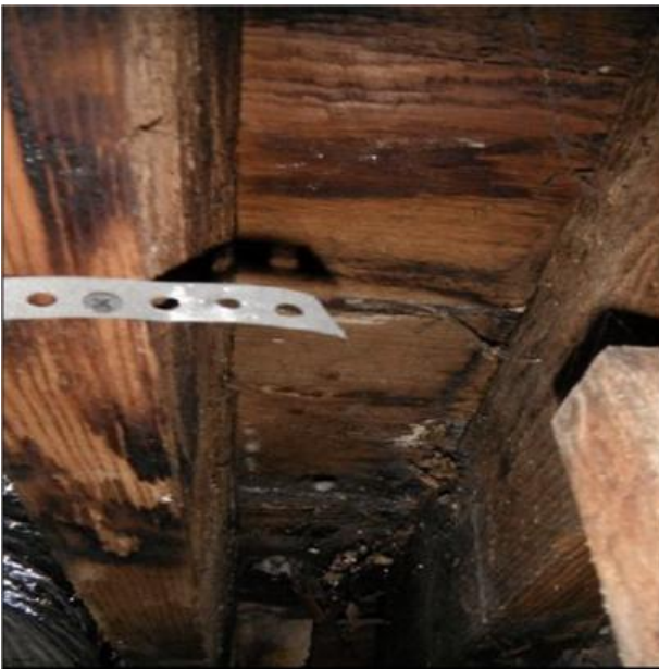
Photo 7 : Fungus damage to framing underneath the entrance stairs
