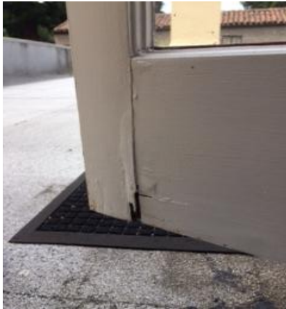
Rot on Window / Door
