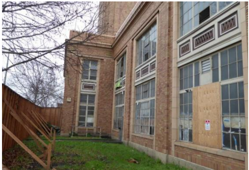
Restoration and reglazing of historic steel windows
