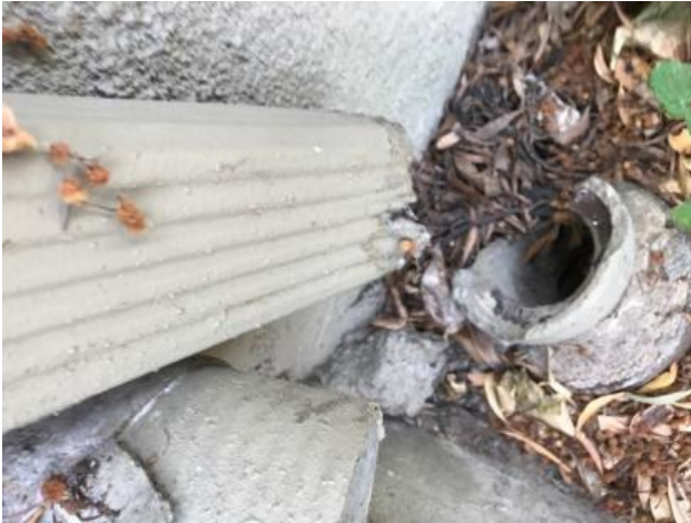
Photo 8: Clay drainage appears to be original
