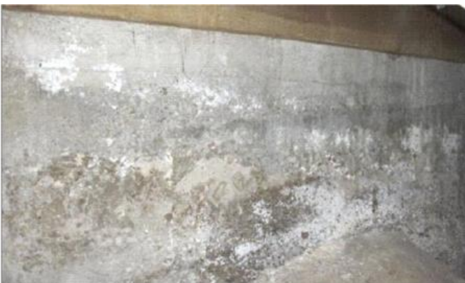
Photo 10: Efflorescence at foundation wall
