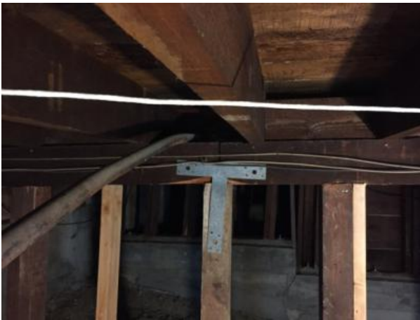
Photo 2: Tilting cripple studs and brace (racked framing)
