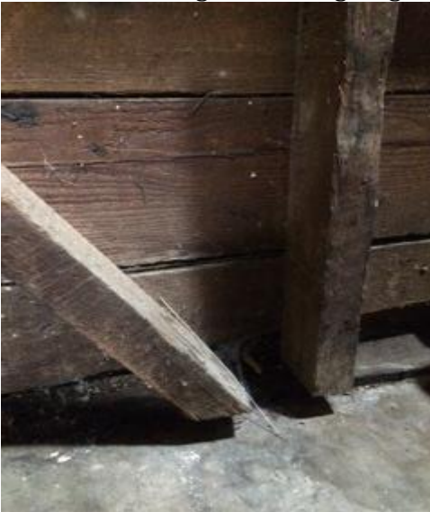
Rear interior garage wall studs Separating from foundation
