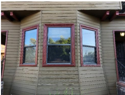
Lower (528) front bay windows
