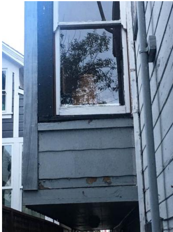
PHOTO C - WORK ITEMS 1-5: Wood window sash with severe dry rot; Asbestos shingles covering original horizontal redwood siding; Visible paint peeling
