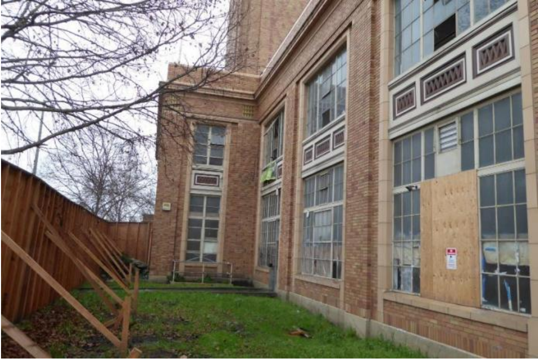
Window restoration and reglazing of historic steel windows on the first two floors of the primary (northeast) facade. Perform visual inspection and repair historic steel windows on first two floors of the primary (northeast) facade as needed. Replace all broken panes of glass and all deteriorated glazing putty. Repaint window sashes and frames.
