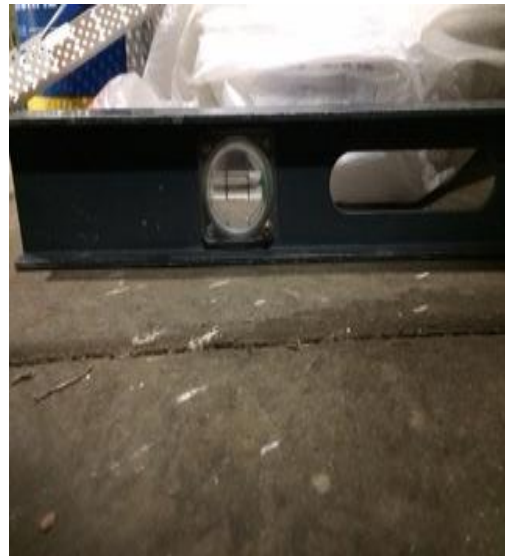
Garage floor warped by Redwood roots The slope is 4" per yard
