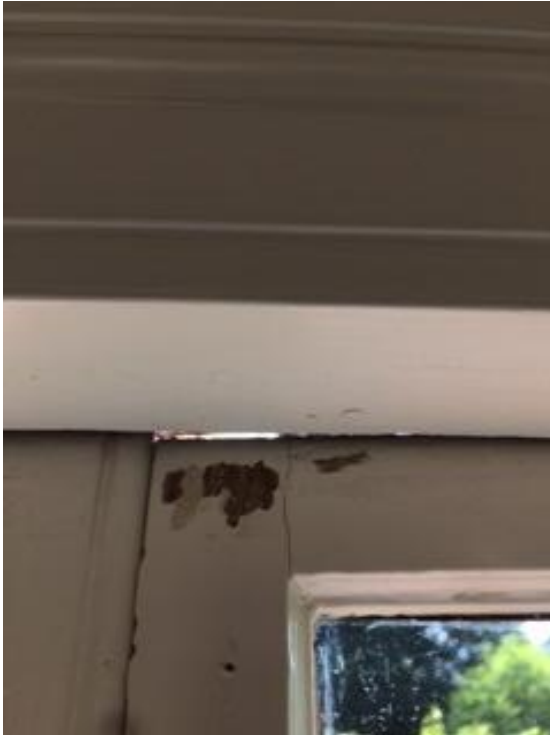
Casement window details of gap and rot
