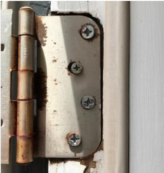
Photo 19: Frame rot on French door due to water intrusion issues
