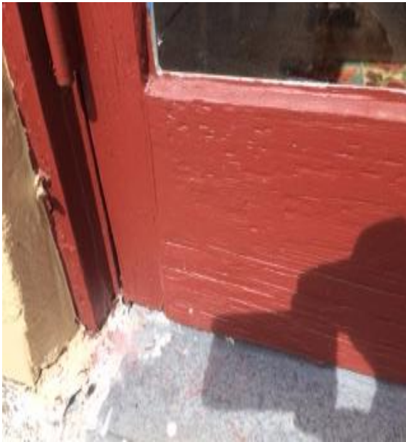
Wood Rot details on door
