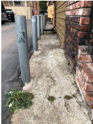
View of west side of house from front
