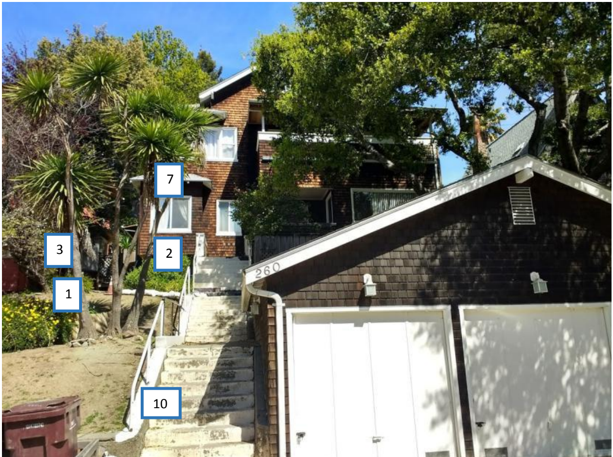
Figure 1: Primary façade from Park View Terrace
