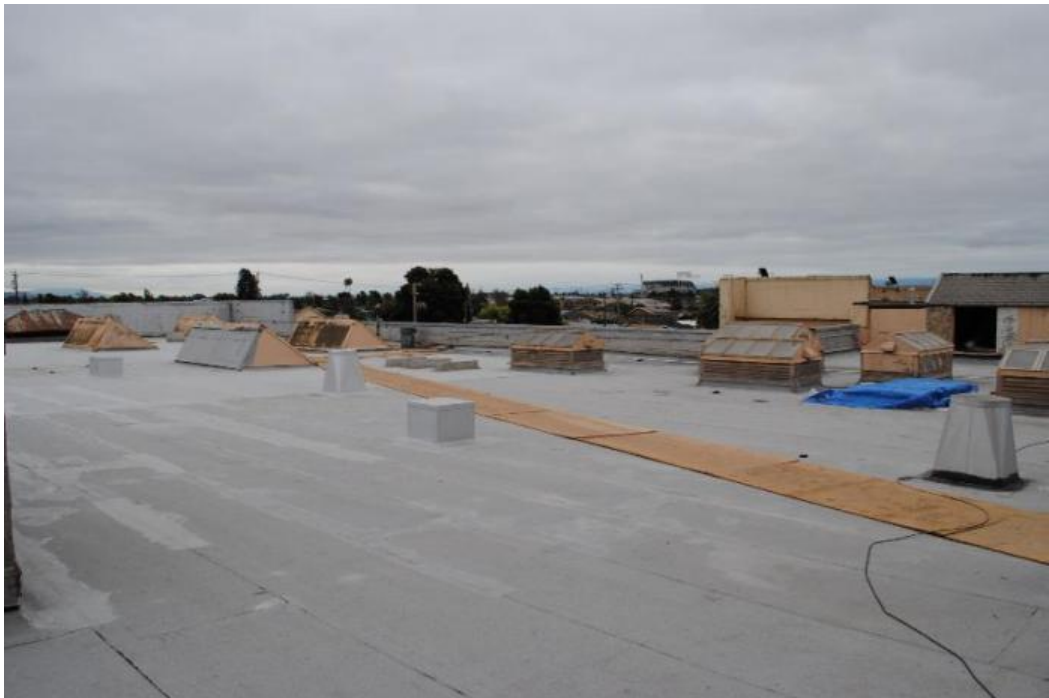
Counter-flashing work at skylight curb connections to roof.
