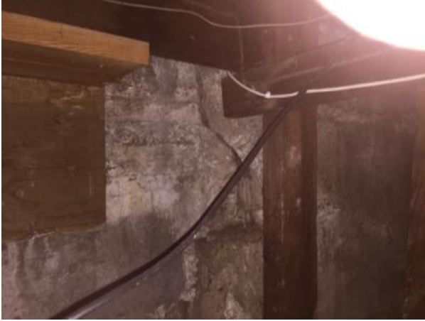
Photo 1: Large crack and crumbling at front foundation near the angled bay window
