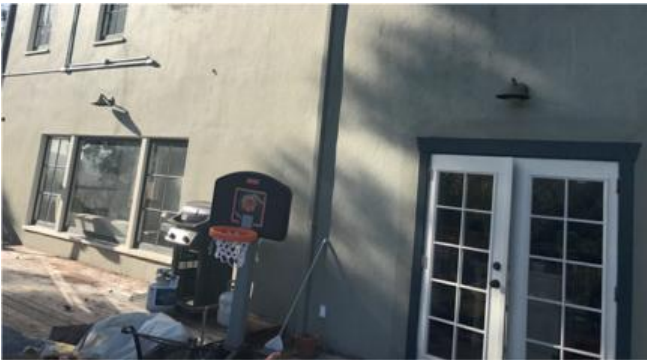
Photo 20: Photo from the deck to show placement of the windows for reference
