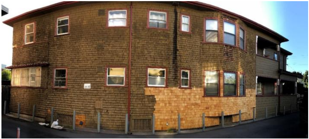
Panoramic view of west side of 528 28 th St
