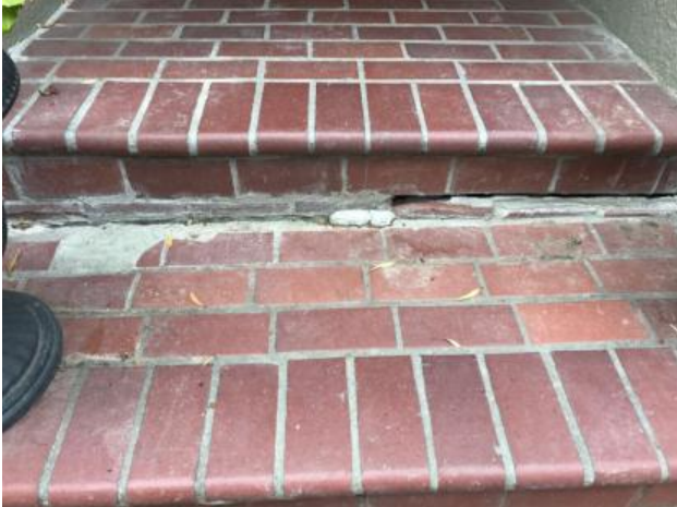
Photo 6: Brick Entrance Stairs Crack
