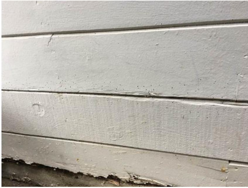
PHOTO E – WORK ITEMS 3-5 – Horizontal siding with severe dry rot and wood beetle damage
