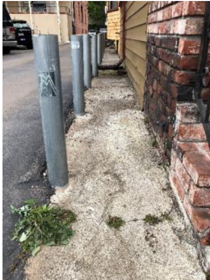
Drainage, west side of house from front
