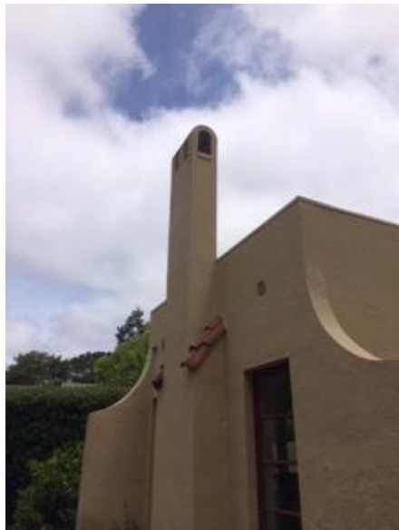
Historic chimney in danger of collapse
