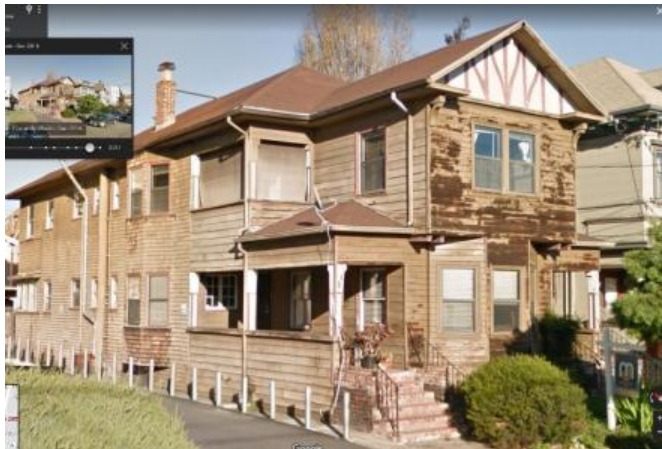
View of 528 28 th St from southwest corner (Dec 2016 – Google Street View)
