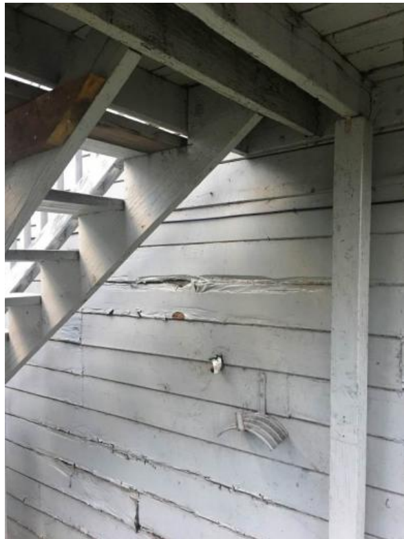
PHOTO D – WORK ITEMS 3-5 – Horizontal siding with severe dry rot, fungus damage and peeling paint
