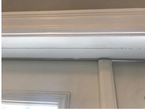
Photo 16: French Door Interior water intrusion
