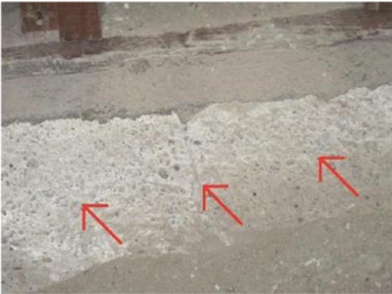
Photo 5: Cracking and spalling
