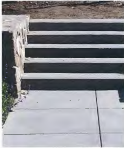
CONCRETE WITH CHEEK WALL
