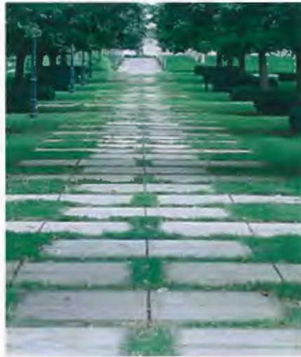
GROUNDCOVER AND PAVERS
