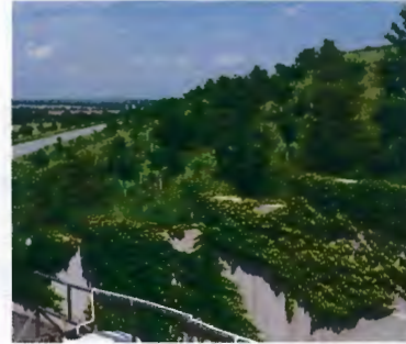
④ RETAINING WALL
