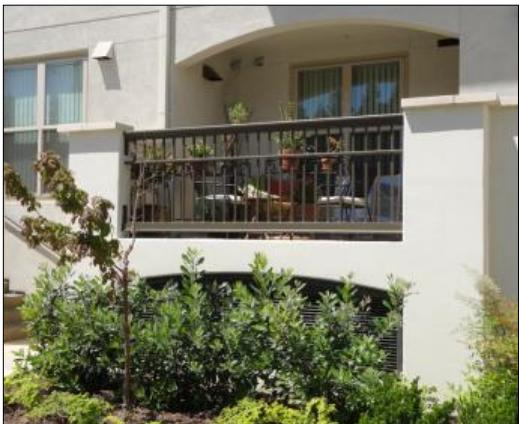
Figure 3.5.e: This parking podium is designed as an integral part of the balcony and screened from the sidewalk by landscaping and a decorative grill.
