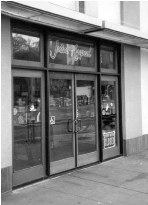
*2.2.3 Doors with one large vertical glass panel and wide wood or metal borders (stiles and rails) are a good choice for almost all ground floor entries. For pre-Art Deco (1930s) ground floors, wood stiles and rails usually work best.*
