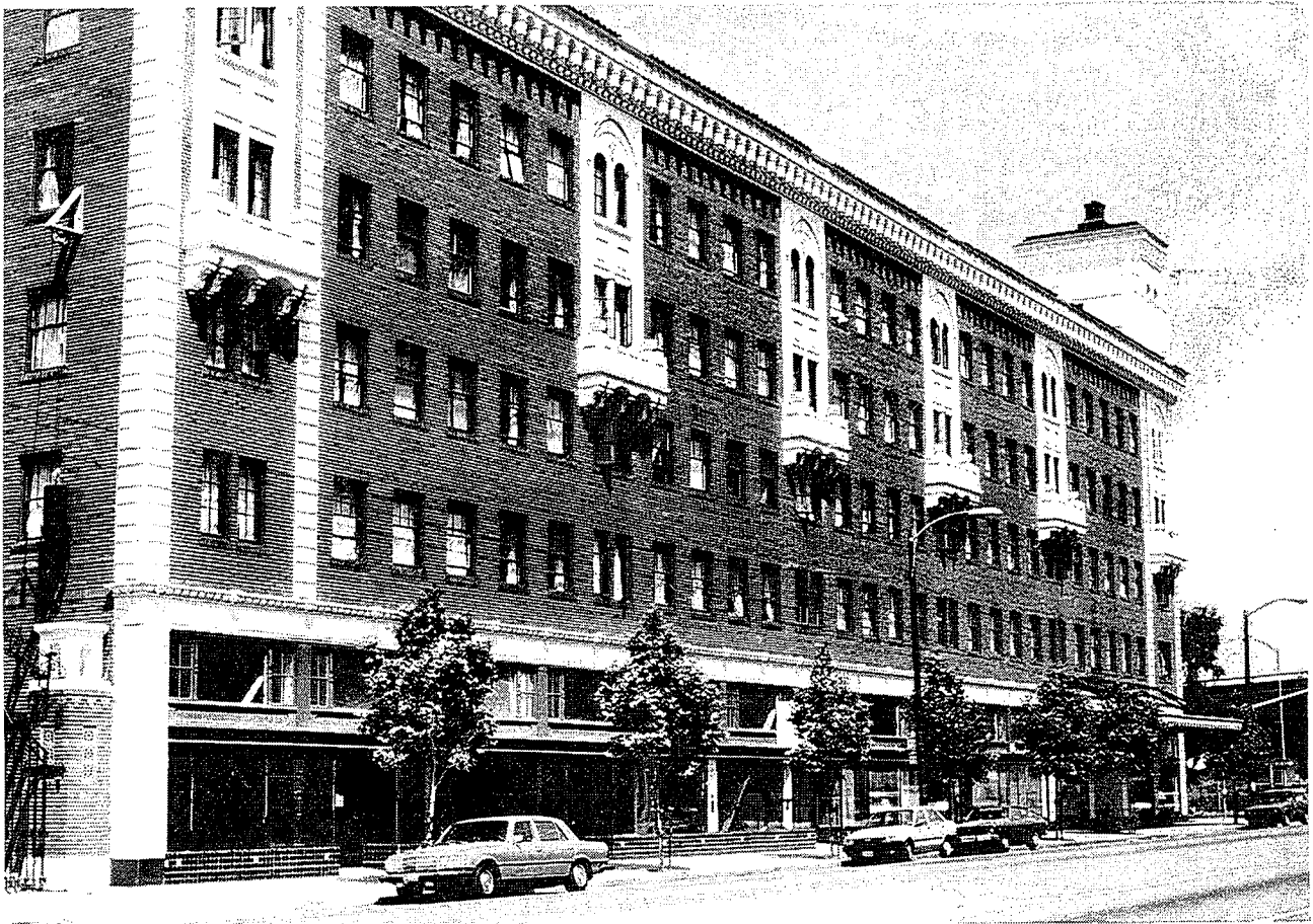
The historic California Hotel on San Pablo Ave. provides for the special housing needs of the neighborhood.
