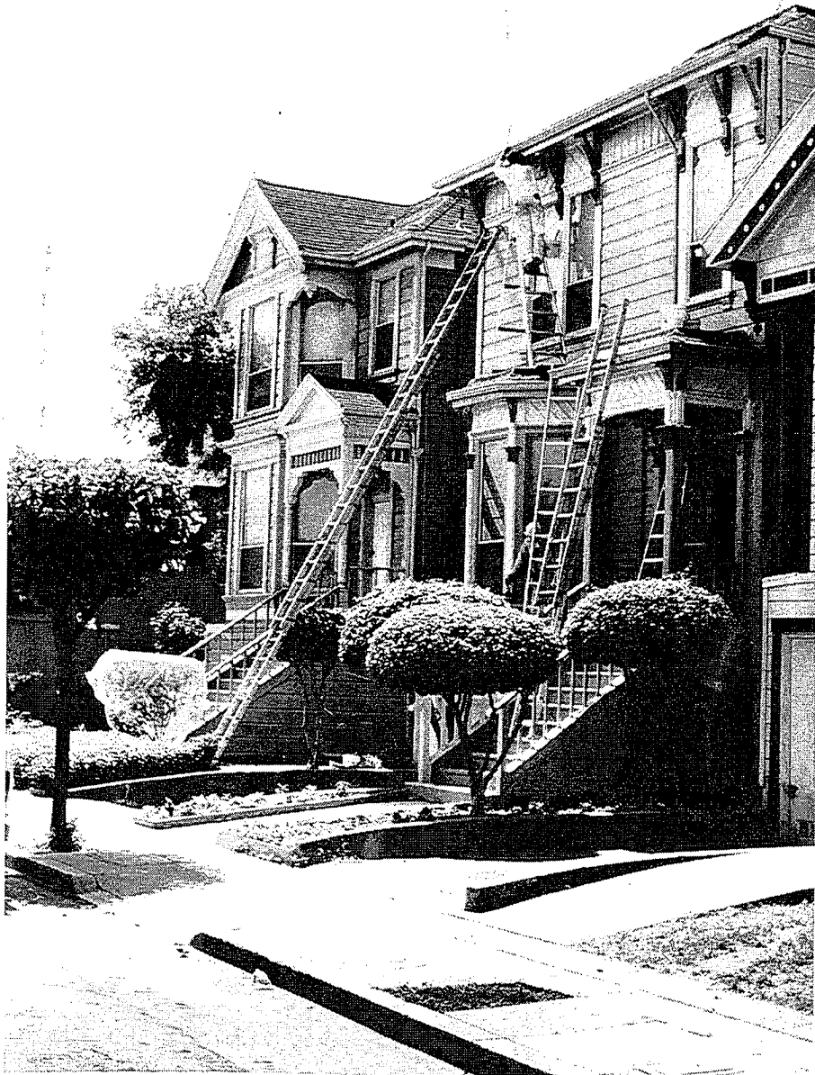
Rehabilitation work being completed on one of the many stately West Oakland Victorians.
