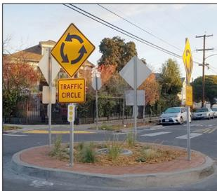
The recently-designated neighborhood bike route (aka bike boulevard) on Plymouth St was enhanced with the addition of nine traffic circles between 81<sup>st</sup> and 103<sup>rd</sup> Aves. The circles were installed to calm traffic and provide greenery along this 1.5-mile route connecting the Eastmont and Elmhurst
