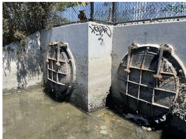
Photo 6: Flap gates on 48" culvert outlet
