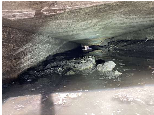
Figure 8 – Catch Basin on Bernhardt Drive (top); Standing Water in Catch Basin (lower left); Sedimented Culvert (lower right)
