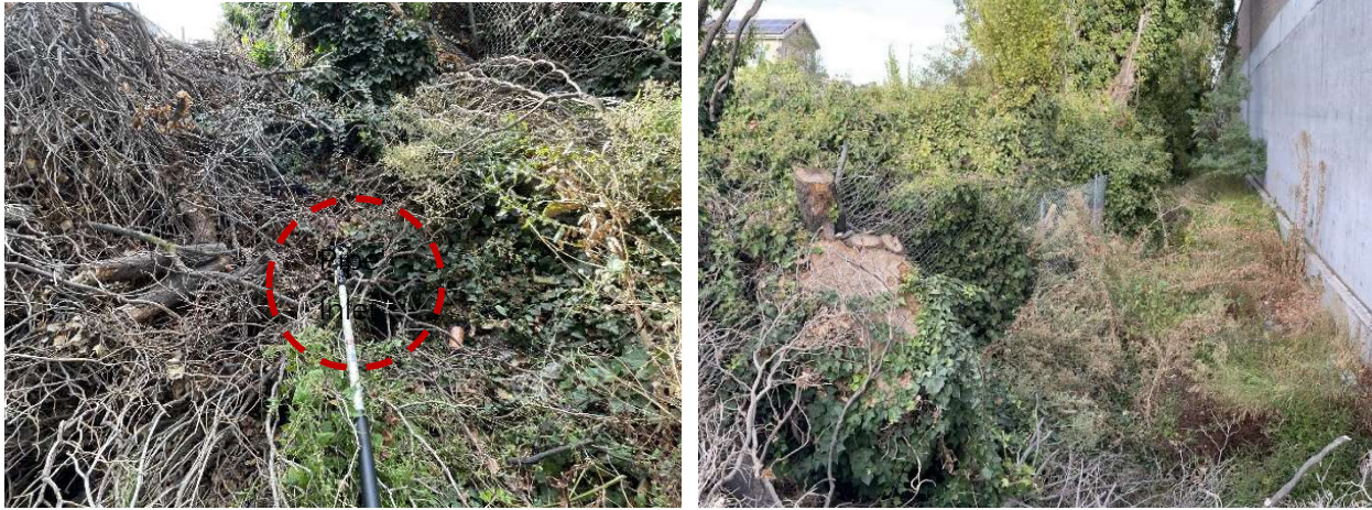
Figure 9 – Overgrown Pipe Inlet (left); Overgrown Channel (right)
