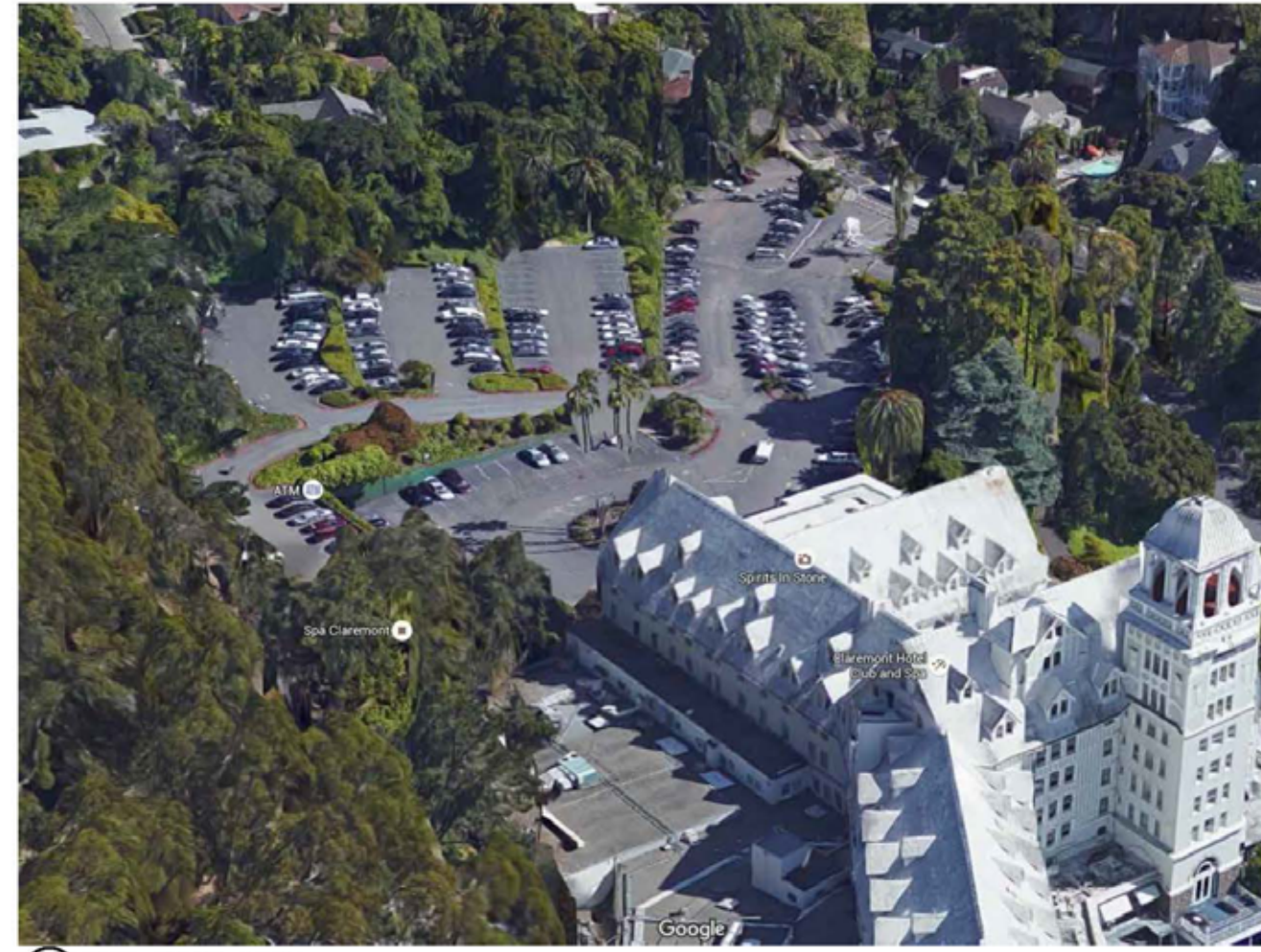
① SITE: AERIAL VIEW
