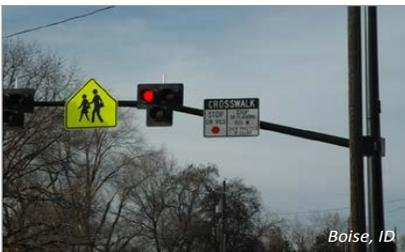
*A pedestrian hybrid beacon is a pedestrian activated display that is unlit when not in use. It begins with a yellow light alerting drivers to slow, and then displays a solid red light requiring drivers to remain stopped while pedestrians cross the street. Finally, the beacon shifts to flashing red lights to indicate motorists may proceed after pedestrians have completed their crossing.*
