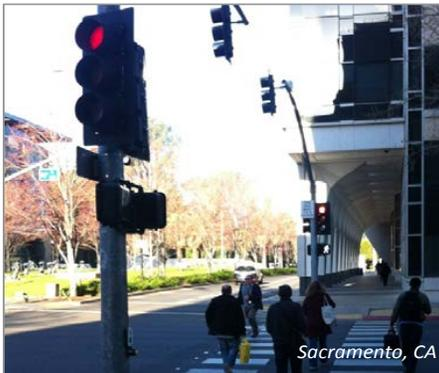
A leading pedestrian interval gives pedestrians a 2-5 second head start before the concurrent vehicle phase turns green to allow pedestrians to enter and occupy the crosswalk before turning vehicles get there.
