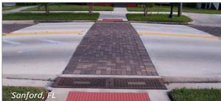
*Raised pedestrian crossings bring the level of the roadway even with the sidewalk, providing a level pedestrian path and requiring vehicles to slow. Raised crossings can be used at midblock crosswalks or intersections.*
