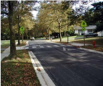
*A pedestrian crossing or intersection area raised vertically to give motorists and pedestrians a better view of the crossing area. A raised crosswalk is essentially a speed table marked and signed for pedestrian crossing.*
