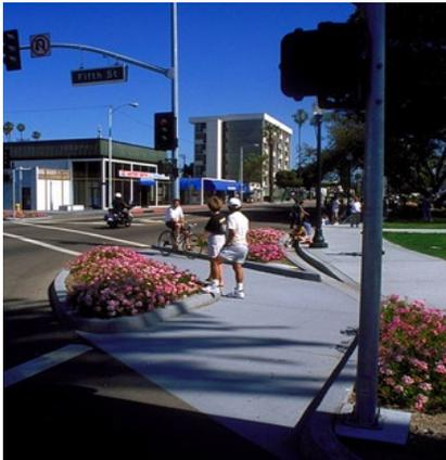
*Reduces right-turning vehicle speeds at an intersection by forcing sharper turns. Reduced corner radii also shorten crossing distances for pedestrians.*
