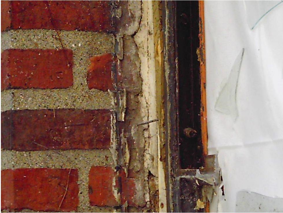
A close-up photograph showing damaged caulk around a window frame. The caulk is dark and appears to be peeling or cracked, revealing the underlying wall material. The window frame is visible on the right side.                         |
