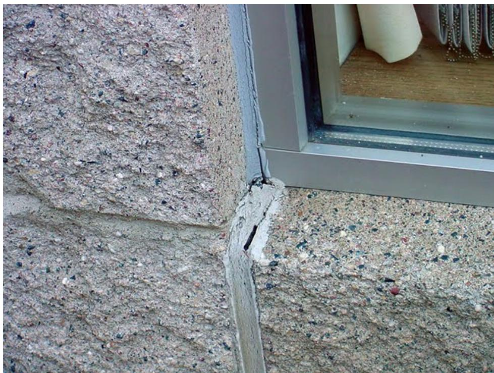
A close-up photograph showing worn and cracked caulk around a window frame. The caulk is light-colored and appears to be peeling or cracking, especially at the bottom edge of the frame. The window frame is visible on the right side. |
