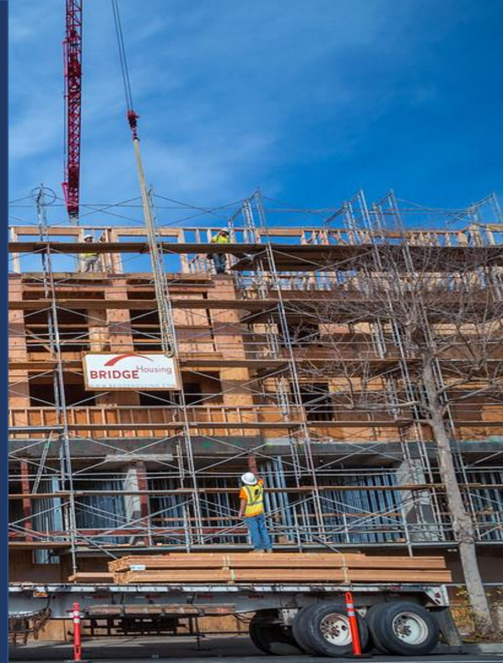
Photo: Greg Linhares, City of Oakland
