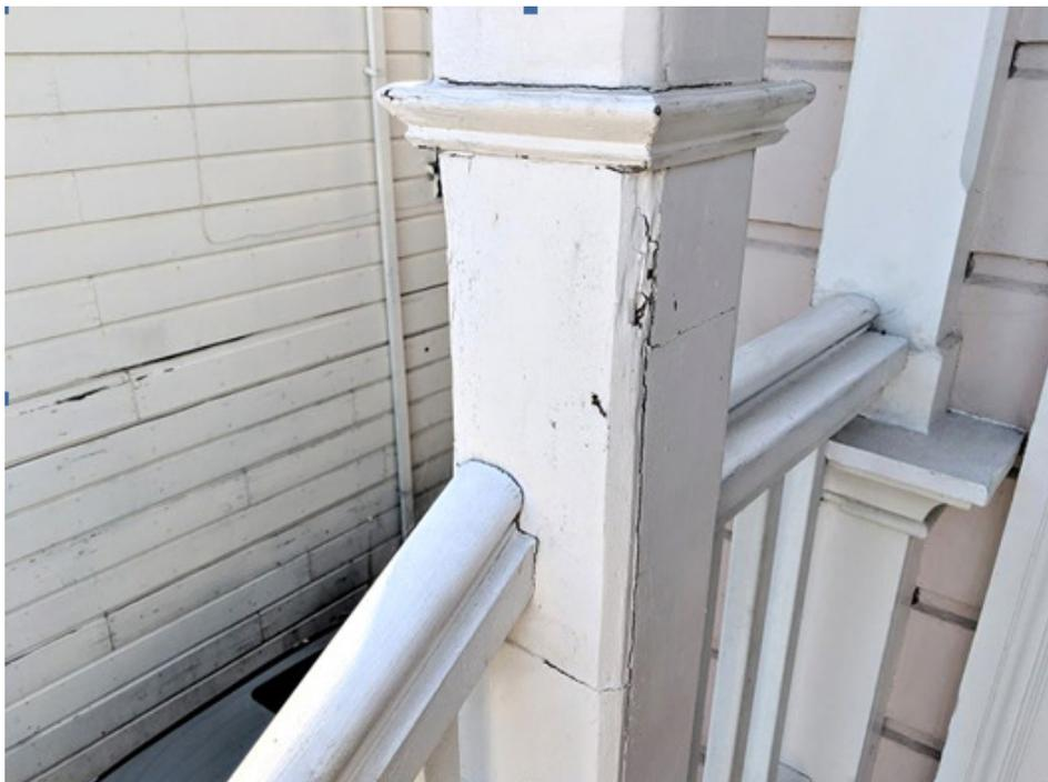
Patched dry rotted square chamfered columns located on the portico porch. They should be replaced with historically accurate turned balustrades.
