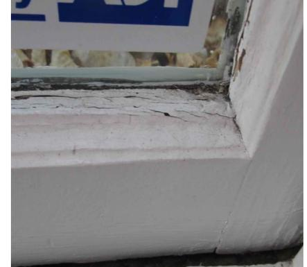
Some wood is dry-rotten but most damage is the result of aging putty, sun exposure and water seepage.
