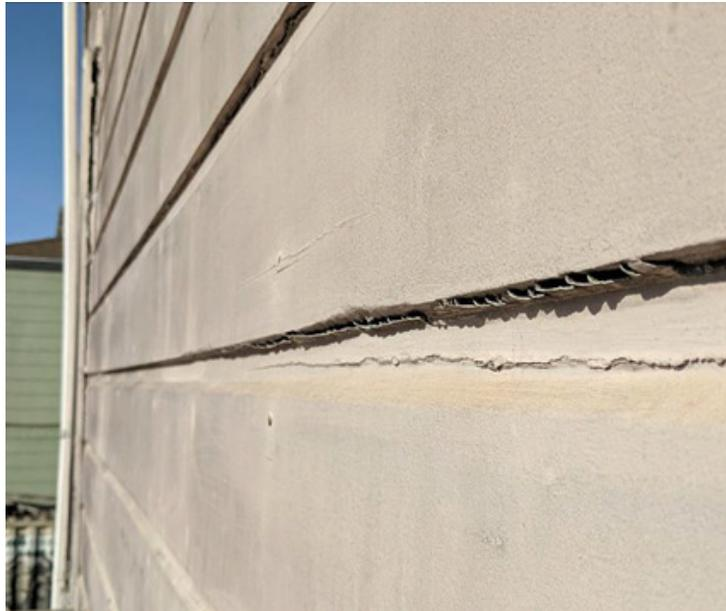
The finish nails are pushing out of the siding in many places and need to be reset (left). The caulking which was added to the bottom edges of all the siding boards needs to be scraped out as it is chipped and blistering, and should not have been placed there in the first place (right). The entire exterior of the house then needs to be re-primed and painted.
