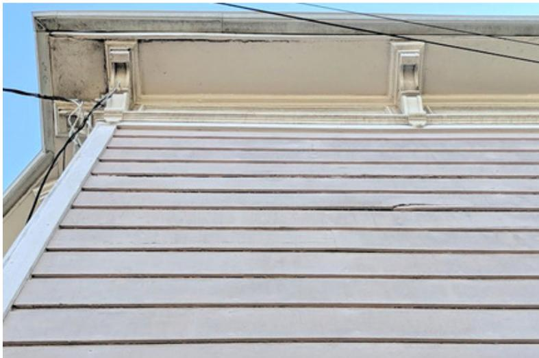
The gutters are cracked and their fastening screws are rusted, which has caused the gutters to detach from the home in many areas. The shingle roof is leaking in various places and also needs to be totally replaced to prevent further damage, and proper ridge and eave ventilation must be added.
