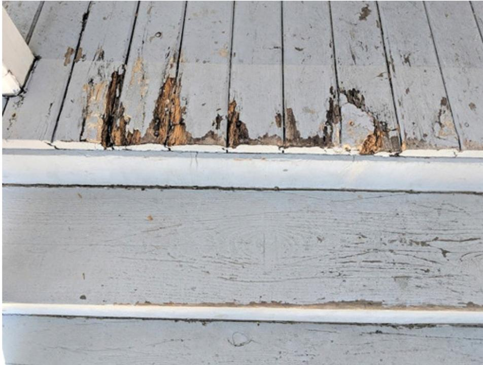
Rotted tongue and groove floor boards located on the front porch.
