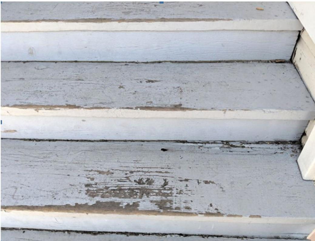
Dry rotted treads on the front staircase.
