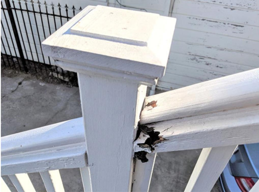
Dry rotted hand rail on the front staircase. Most of the structure is rotted, and so the entire front staircase needs to be rebuilt.
