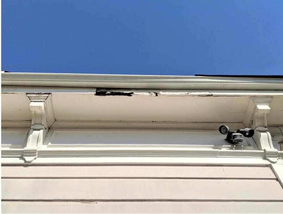
Due to the water entering the eaves, the fascia, soffits and rafter tails are dry rotted on all four sides of the house. A number of the decorative brackets are also dry rotted and need to be repaired or replaced.
