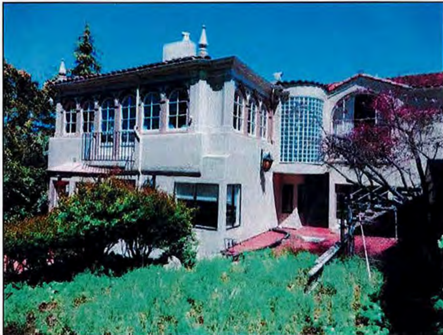
Figure 5. Overview of south façade, view north (SWCA, 2018).
