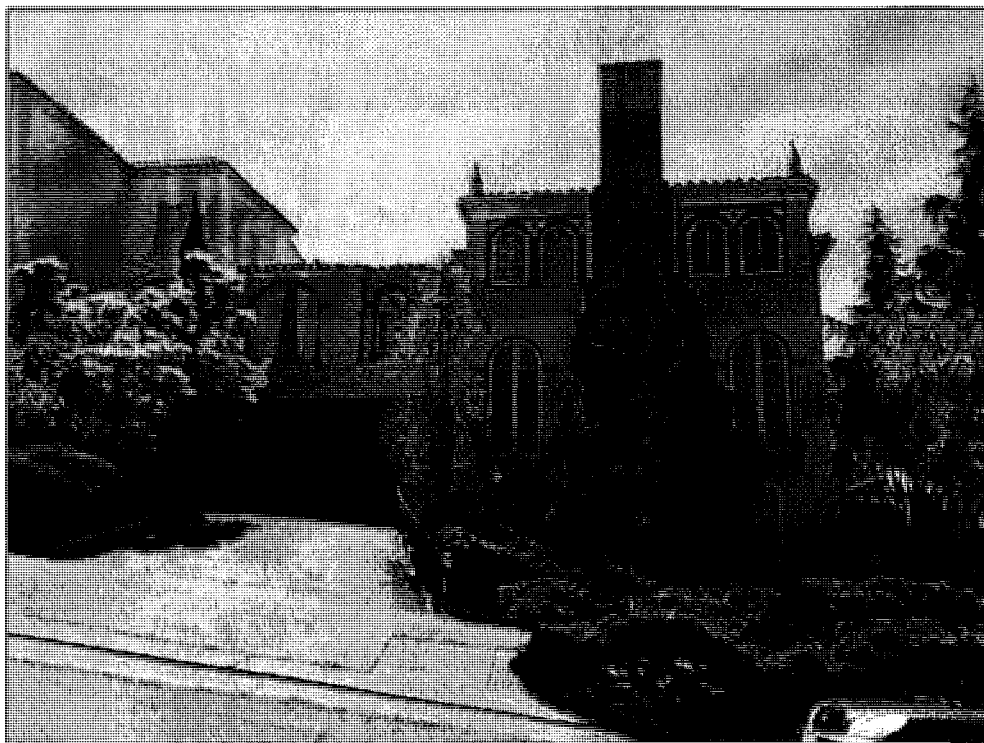
Figure 14. Overview of north façade, view south (SWCA, 2018).
