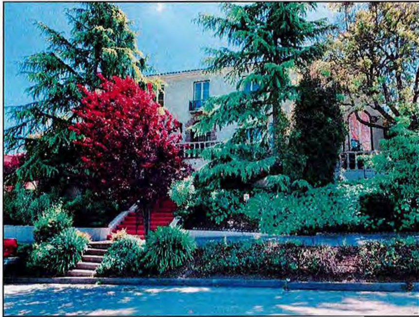
Figure 2. Overview of primary (west) façade at 664 Haddon Road, view east (SWCA, 2019).
