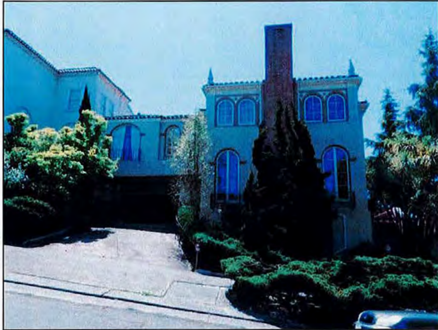
Figure 4. Overview of north façade, view south (SWCA, 2018).
