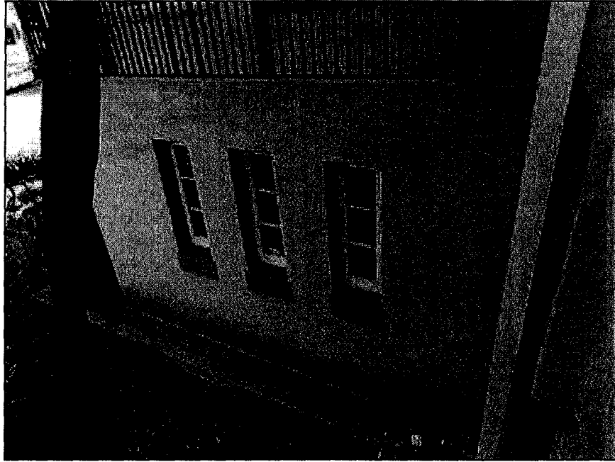
Figure 6. Detail of basement level left of staircase on primary (west) façade, view northeast (SWCA, 2018).
