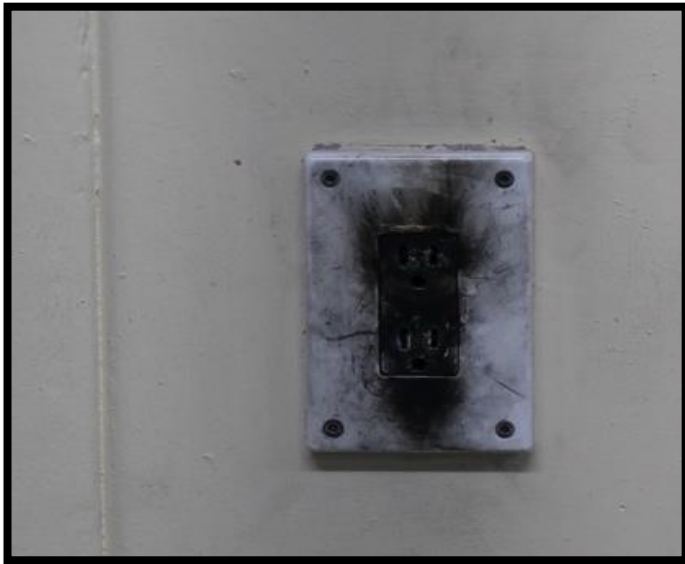
Damaged electrical outlet in housing unit
