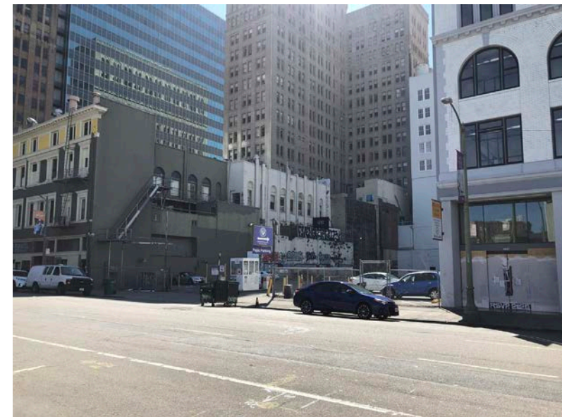
3 - View towards site from east
