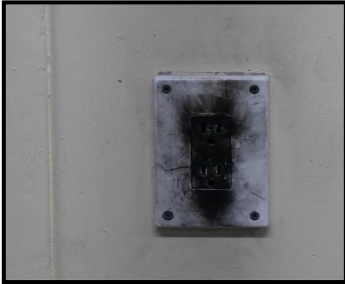
Damaged electrical outlet in housing unit
