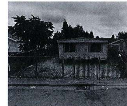
330 105th AVE - RESIDENCE
