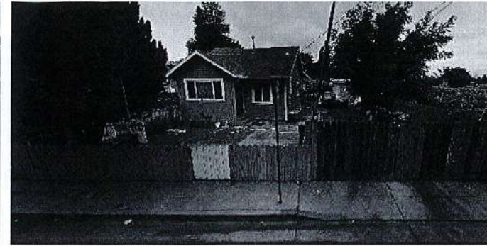
309 105th AVE - RESIDENCE
