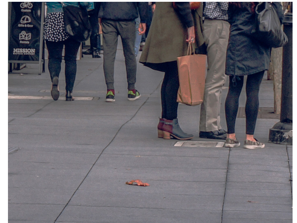
INTEGRAL COLOR CONCRETE SIDEWALK
