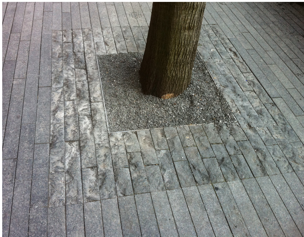
PAVER-COVERED TREE GRATE AT PLANTING TRENCH
