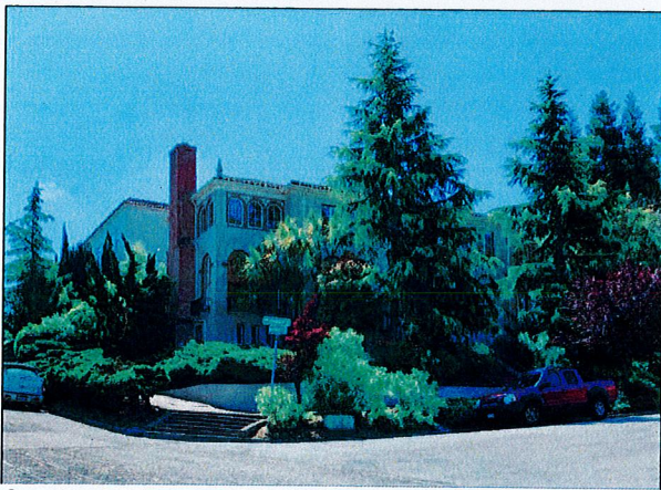
Overview of north and primary (west) façade at 664 Haddon Road, view east (SWCA, 2019).
