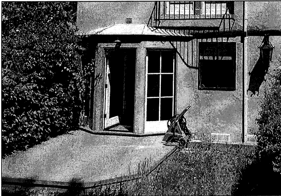
Figure 65. Detail of patio of breakfast room, view north (SWCA, 2018).
