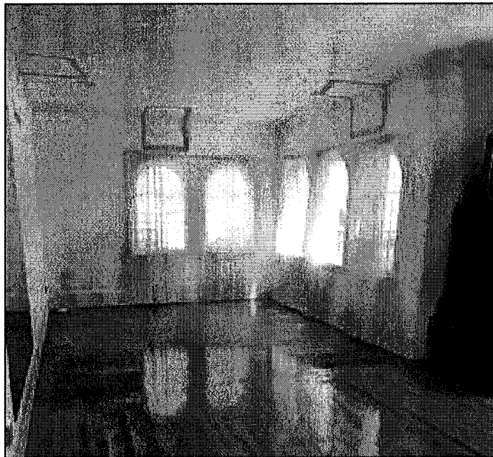
Figure 46. Northeast bedroom, view northeast (SWCA, 2018).
