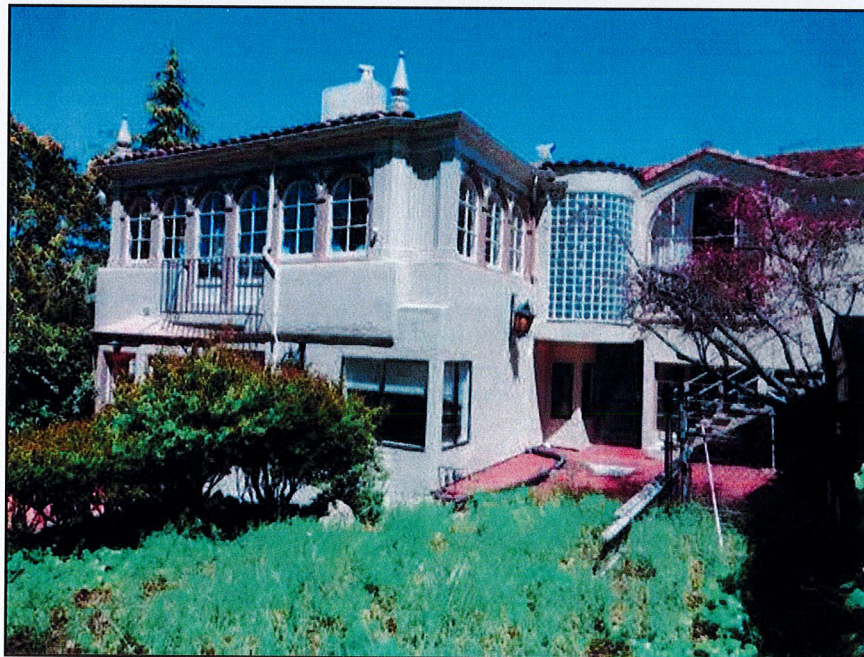
Figure 5. Overview of south façade, view north (SWCA, 2018).
