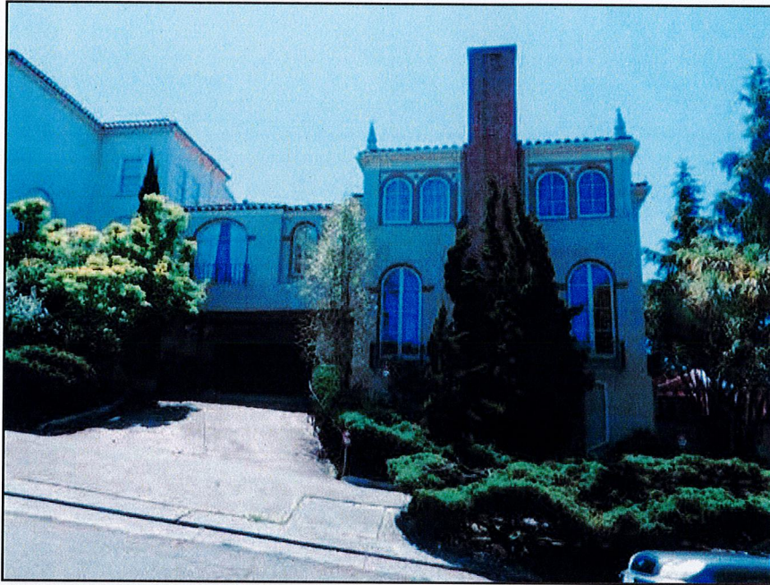
Figure 4. Overview of north façade, view south (SWCA, 2018).
