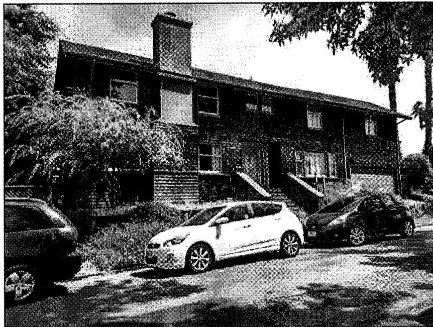
Figure 76. 662 Kenwyn Road, view southeast. Designed by Charles W. Dickey, constructed 1914 (SWCA, 2018).
