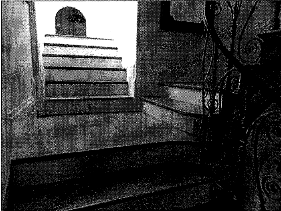
Figure 44. Second-floor landings, view east (SWCA, 2018).
