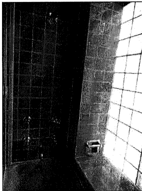
Figure 48. Hallway bathroom, view northeast (SWCA, 2018).
