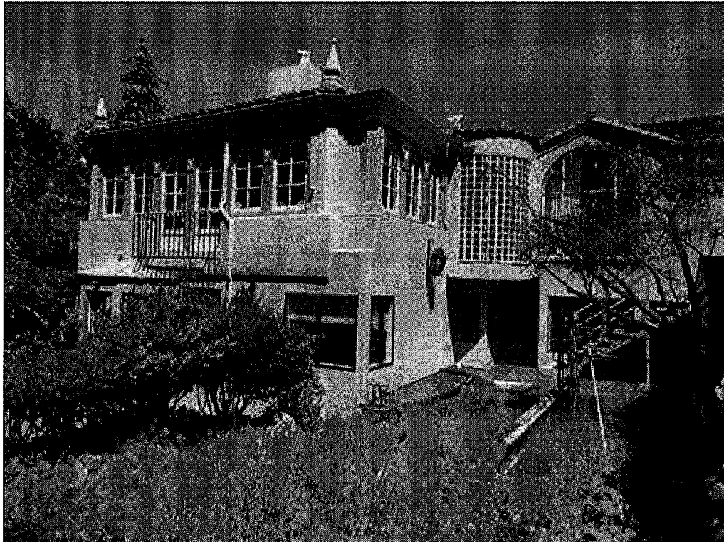
Figure 22. Overview of south façade, view north (SWCA, 2018).
