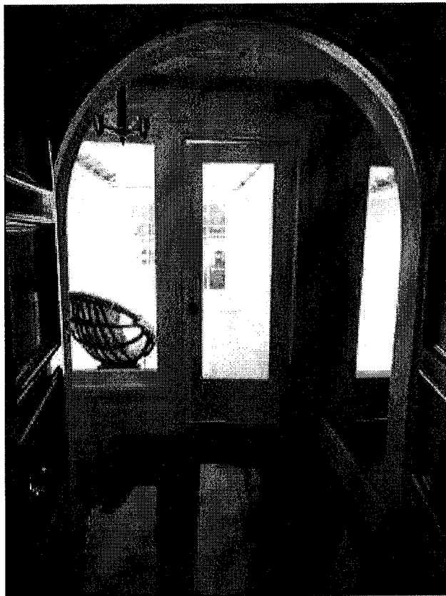
Figure 60. Back (east) end of stair landing, view north from library (SWCA, 2018).
