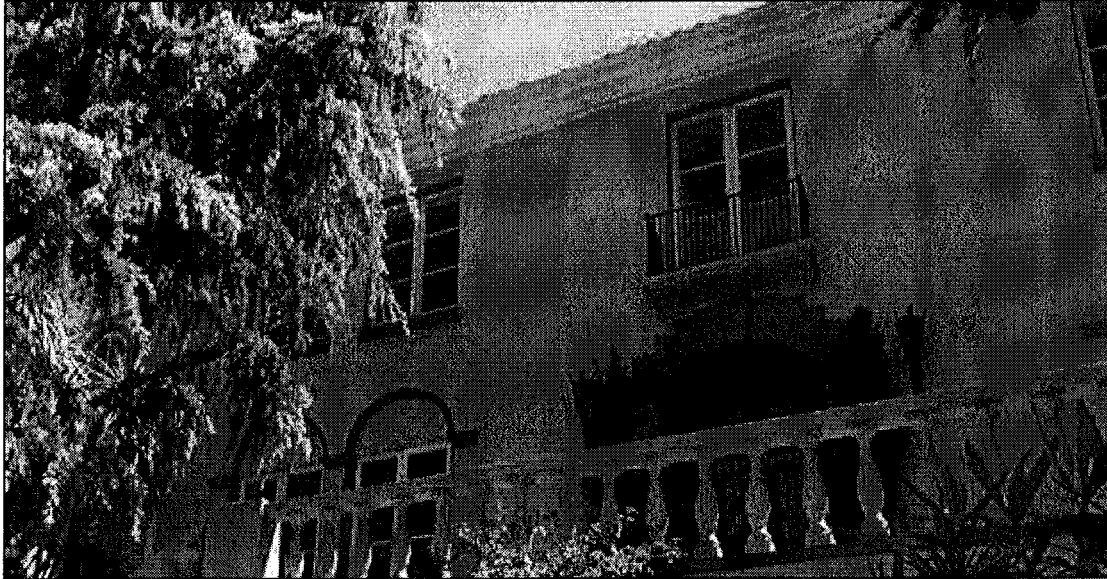
Figure 12. Detail of second-floor windows, view east (SWCA, 2018).
