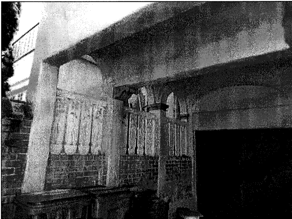
Figure 21. Detail of perimeter wall at east boundary, ceiling in front of garage and garage door, view southeast (SWCA, 2018).
