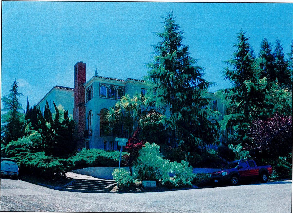
Figure 1. Overview of north and primary (west) façade at 664 Haddon Road, view east (SWCA, 2019).
