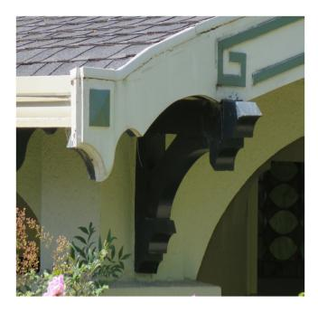
Wood works on trims and barge needs repairs. The paint is peeling and trim is getting damaged
