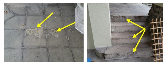
Concrete spalling on the front porch requires re-surfacing Spalling and cracking in the front porch entry requires repair
