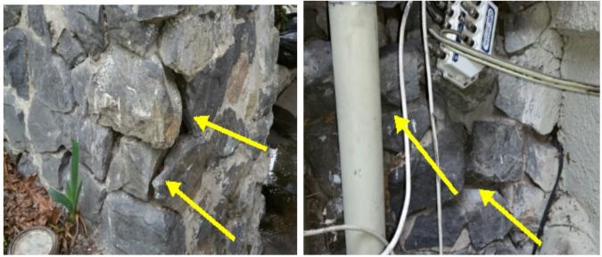
Water Intrusion in the basement in May 2017. Water intrusion in rainy months are severe and requires repair
