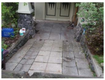
Cracks in concrete driveway seems like causing water intrusion to the basements. Concrete driveway requires repair or resurfacing.
