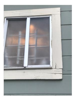
double pane restorative, preferably wood, energy efficient and/or cost-saving windows (upstairs) Replace broken glass, scrape, surface preparation, repaint, re-caulk, repair all windows on front elevations. Replace jalousie window at kitchen with new double-hinge. (see above)
