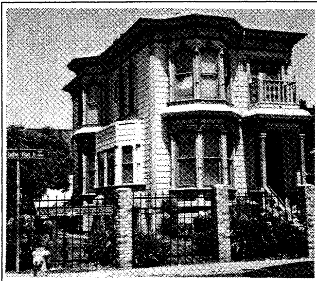
Hanifin House, 1807 Martin Luther King, Jr. Way. Potential Class 2 Landmark adversely remodeled with City assistance. Would probably have been potential Class 1 Landmark prior to remodeling.
