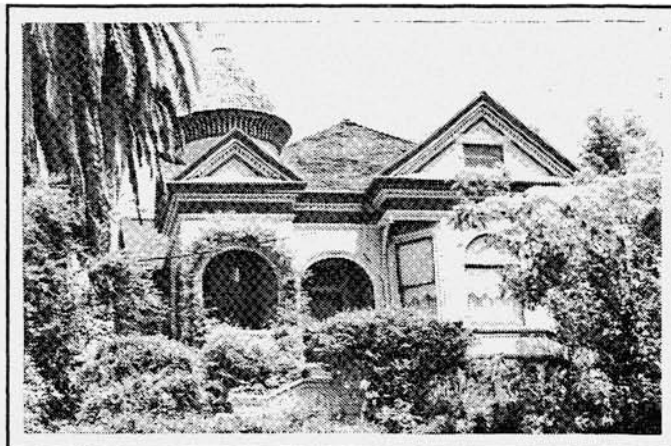
Possible Class 3 Landmark: Saxtorph House, 1937 8th Avenue. Oakland Landmark No. 105. Possible "B" under Landmark Eligibility Guidelines. Does not appear individually eligible for National Register.
