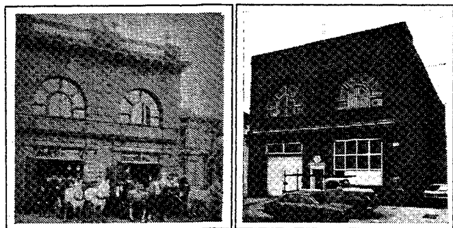
Former Oakland Point Firehouse, 1681 8th Street. Oakland Landmark No. 37. Left: As originally built. Right: Present appearance with cornice, parapet and other detailing removed. Doors also replaced.
