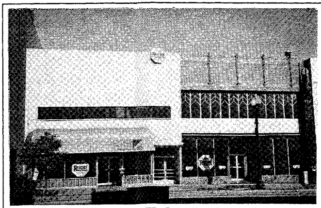
Bowles Building, 1713-21 Broadway/1712-20 Telegraph Avenue. Right side with original Art Deco terra cotta upper floor. Left side covered with stucco. Window shapes also changed.
