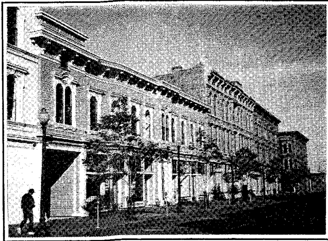
Possible Class 1 Preservation District: Old Oakland S-7 Zone. Area of Primary Importance identified by Intensive Survey. Eligible for National Register of Historic Places.
