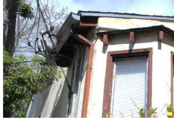
Figure 72. Overhanging eave with exposed rafters and rafter tails at the southeast corner of the original volume, looking north.
