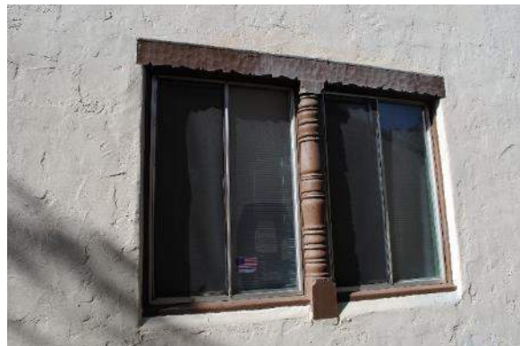
Figure 40. Paired typical windows with a carved wood lintel and central turned wood column at the north end of the northeast façade at the first story.
