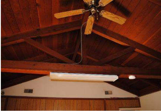
Figure 86. Exposed roof truss of the 1954 addition.
