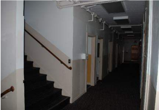
Figure 66. Shifted double-loaded corridor and new staircase at the first story.
