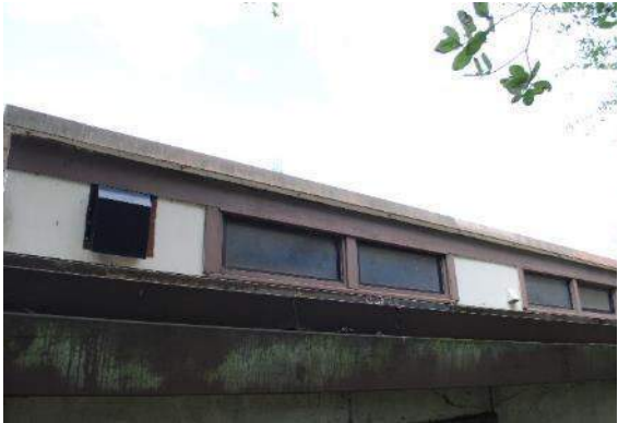
Figure 105. Shed-roofed clerestory windows at the east side of the south wing of Building 6, looking northwest.
