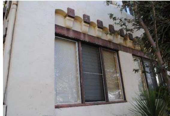
Figure 27. First story windows at the north end of the primary façade, featuring a carved wood lintel and corbeling.
