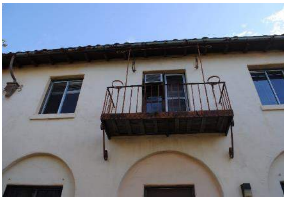
Figure 32. Central balconette at a door opening with non-original windows, above the primary entrance.
