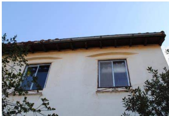
Figure 33. Typical windows with eyebrow openings and sills with terra cotta coping and metal railings.
