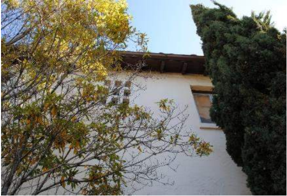
Figure 55. Gridded wood and plaster grille and typical window at the north end of the primary façade at the second story.
