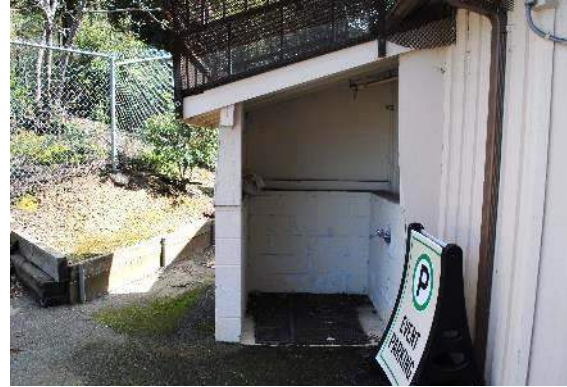
Figure 123. Exterior can wash sink, enclosed by three walls and a shed roof, looking east.
