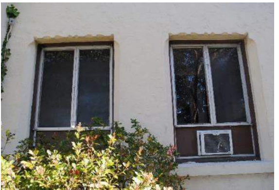
Figure 53. Typical windows with cement asbestos spandrels.
