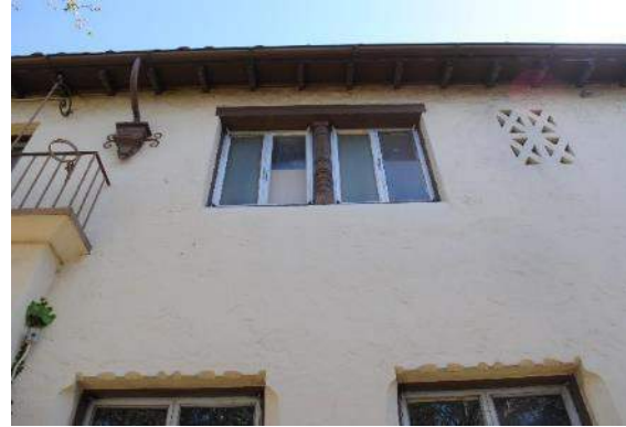
Figure 56. Paired typical windows with carved wood lintel and central turned wood column, and a typical wood and plaster grille at the south end of the primary façade at the second story.
