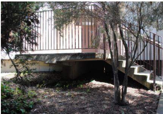
Figure 97. Floating concrete steps and cantilevered concrete entry patio at the primary façade of Building 6, looking east.
