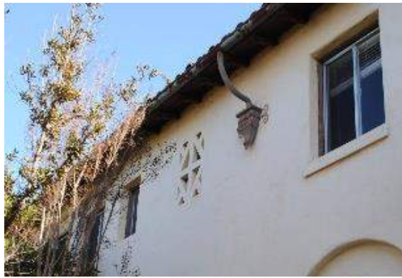
Figure 31. Typical small window, typical wood and plaster grille, and a typical window at the second story.
