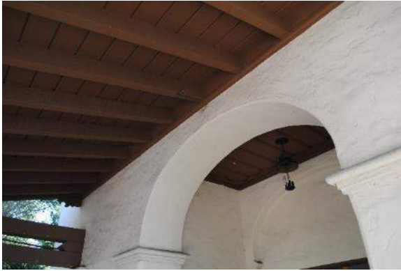
Figure 4. Exposed rafters and wood sheathing of the entry porch roof.
