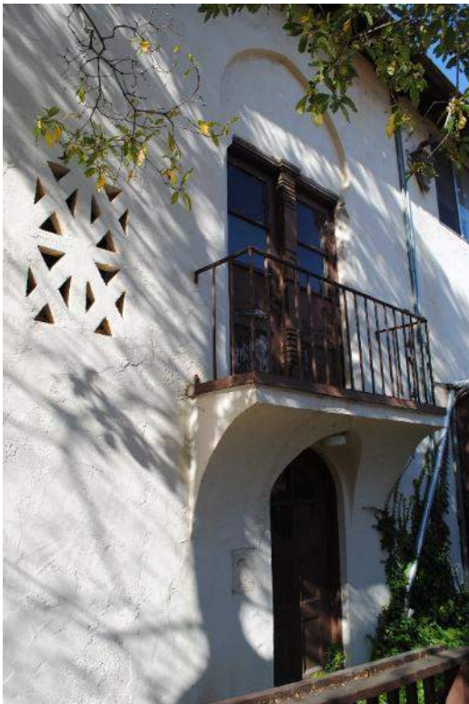
Figure 38. Central arched door at first story, and balconette and pointed horseshoe arch above the paired doors above, looking west.
