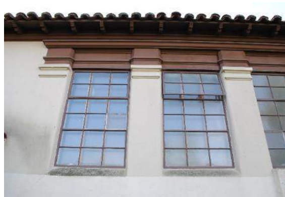
Figure 12. Pilasters, overhanging eaves, and wood cornice at the northwest façade.
