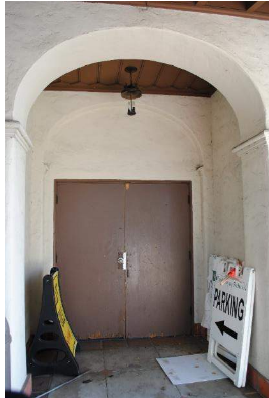
Figure 5. Replacement primary entry doors at a recessed entryway with an arched opening.
