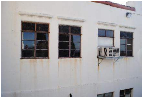
Figure 8. Molded lintels above the windows on the primary façade of the south wing, looking east.
