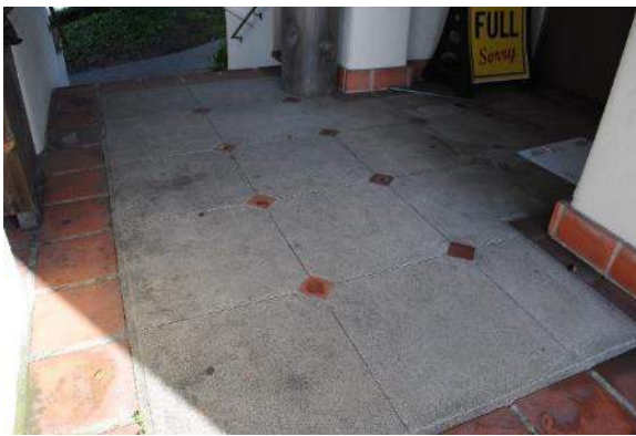
Figure 6. Concrete entry porch with terra cotta tile edging and diamond patterning.
