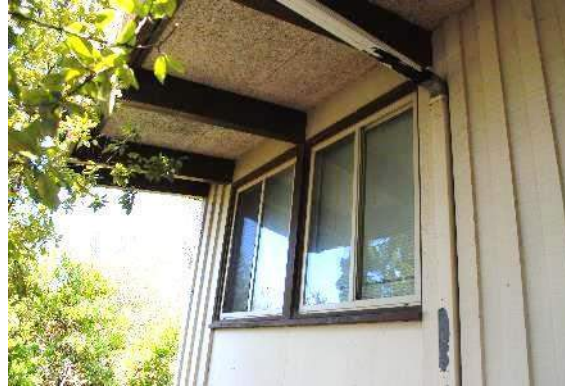
Figure 100. Paired typical windows at the north end of Building 6 with typical board and batten and cement asbestos siding, looking north.
