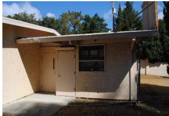
Figure 134. 1963 addition to Building 8 with a low-pitch gable roof with a lower ridge height, looking northeast.
