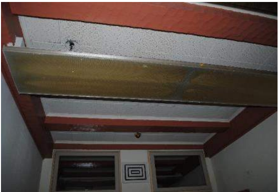
Figure 46. Remaining wood beams in the ceiling of one room on the first floor.
