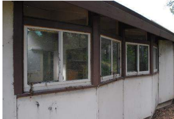
Figure 106. Accordion wall along east façade of south wing, looking northwest.
