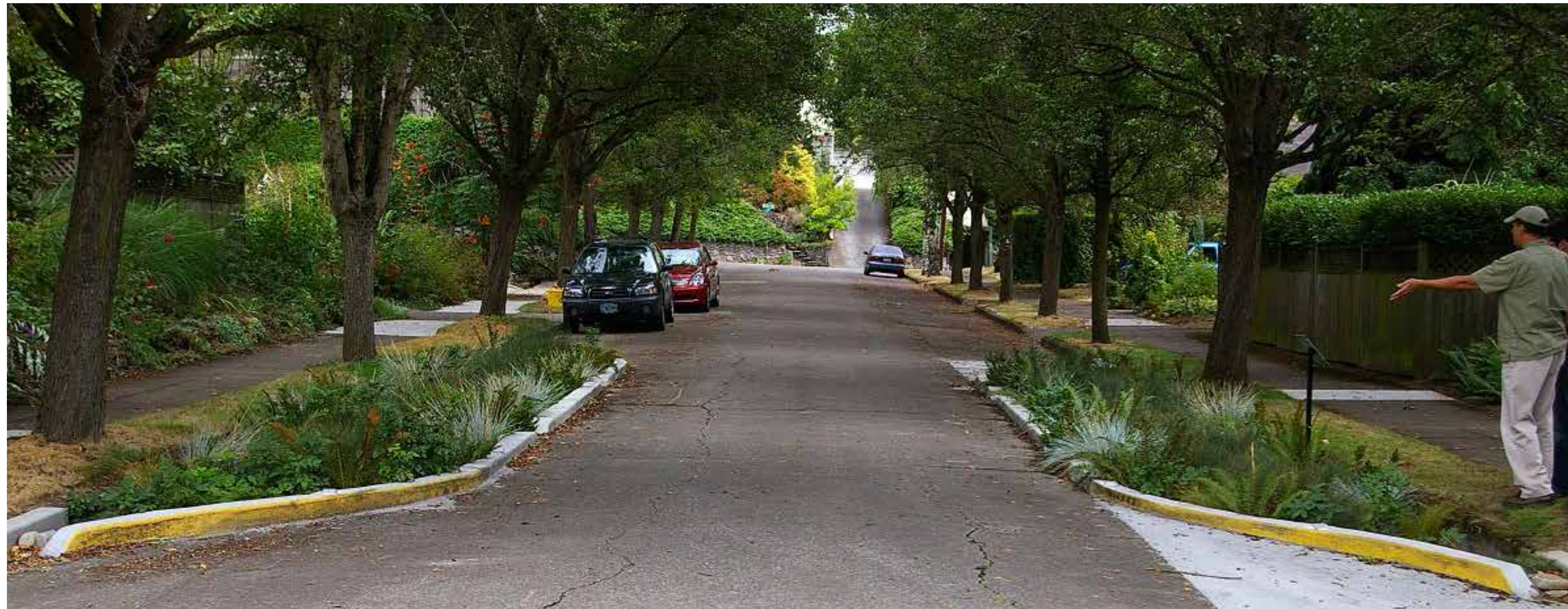
Typical Flow-through Planter / Rain Garden Concept Image
