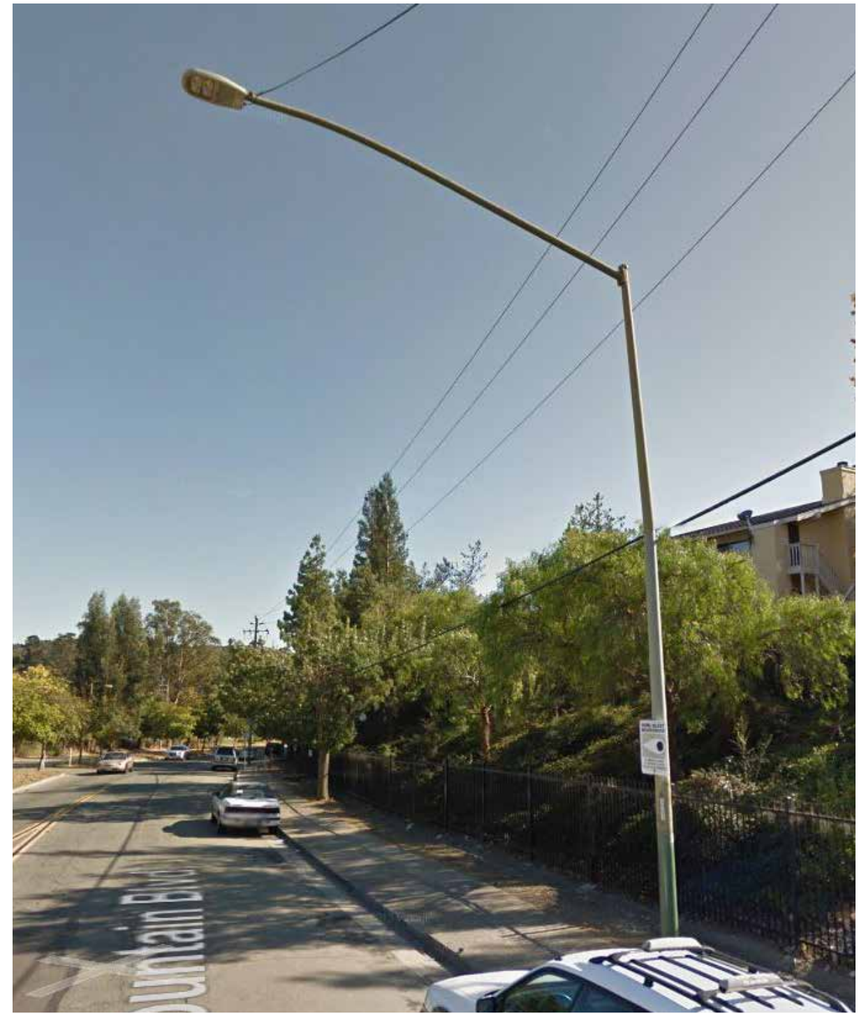
Existing Cobra Head Street Lighting to remain on west side; east side entries only
