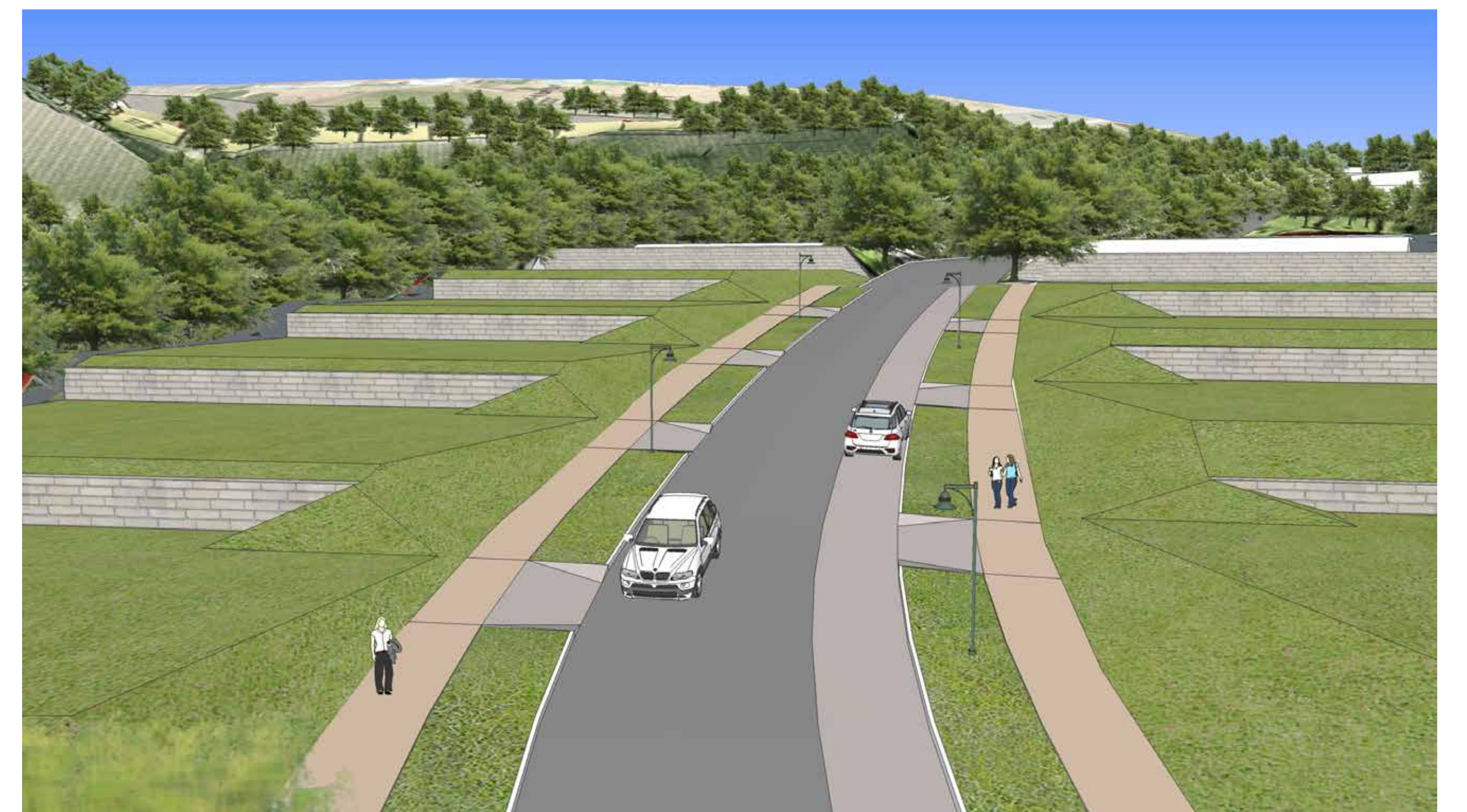
Side Yard Lot Retaining Walls in FDP delivered condition
