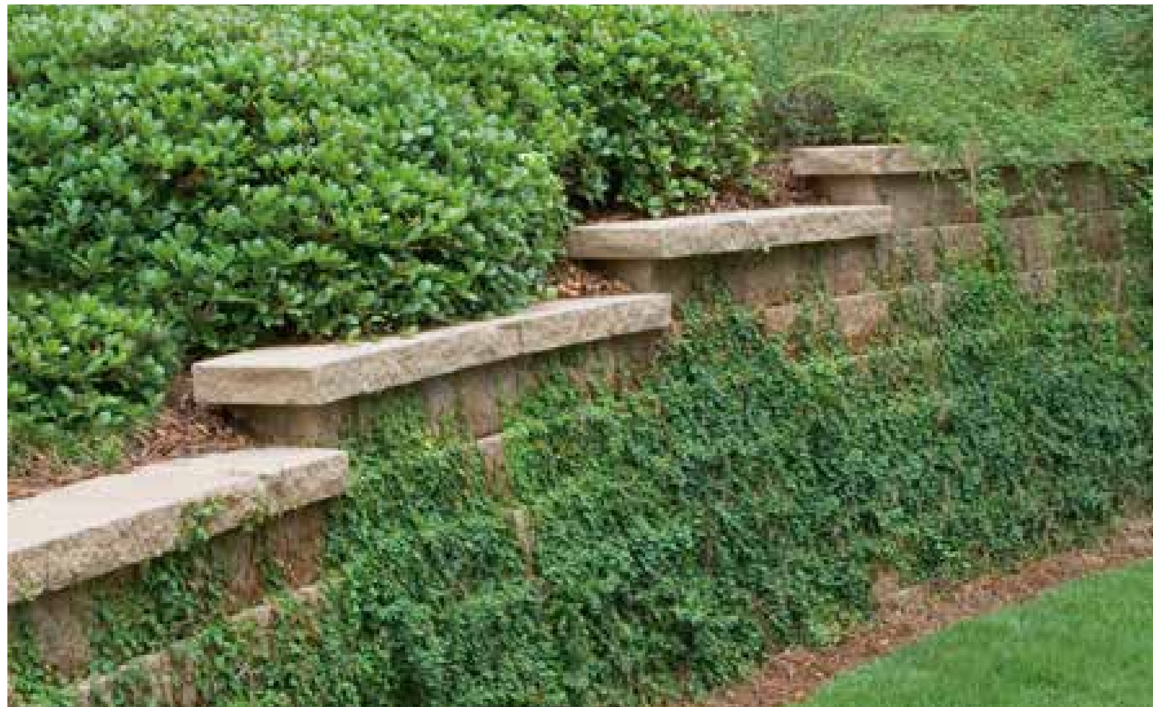
Pavestone 'Anchor Diamond Pro' retaining walls. Straight face style, Sandstone Blend color with vine plantings. Site walls shown on VTTM Sheets C.5.0 - C5.5.
