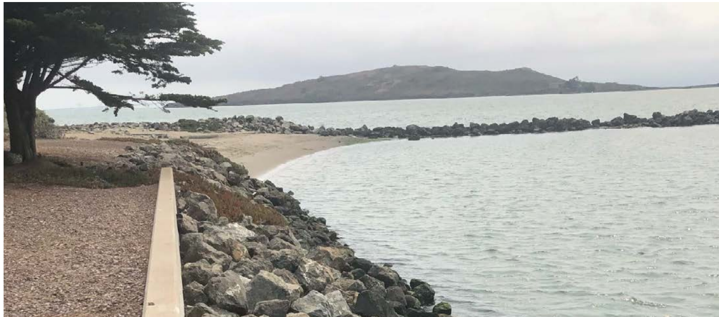
Pocket Beach + Seat Wall and Armoring Integration
