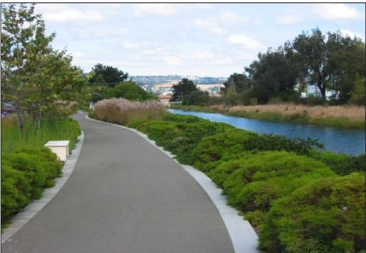
► *Figure 3.9.e: Asphalt is allowable if contained within flush Portland Cement headers. Provide attractive landscaping along the edges of the Bay Trail pathway wherever practicable.*
