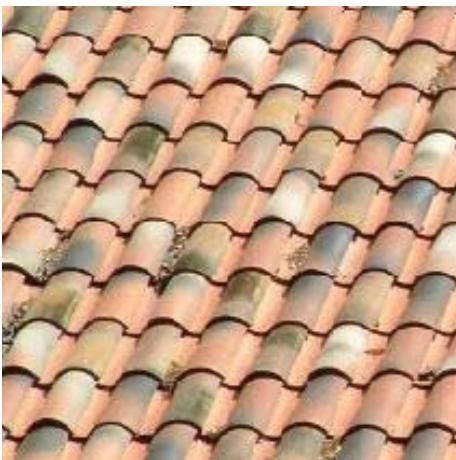
CLAY TILE ROOF
