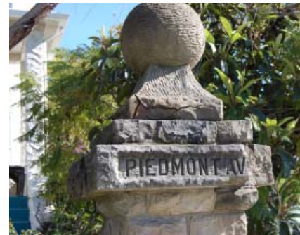
Stone Neighborhood Entry Piers
