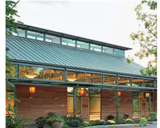
Clerestory windows and natural lighting
