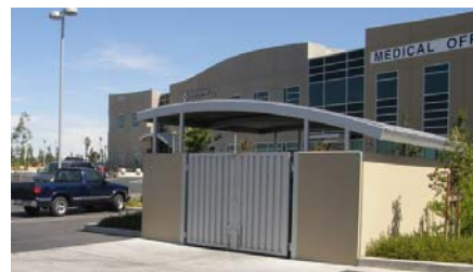
Example of trash enclosure with roof shape related to roof shape of primary building
