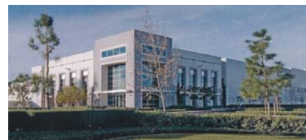
Example of identifiable main entry
