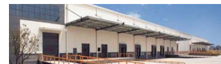
Example of truck docks with awnings
