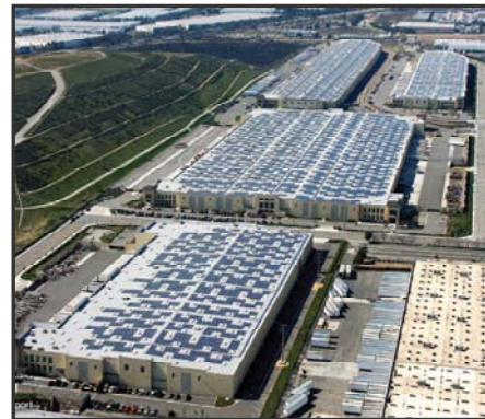
Example of rooftop solar panels
