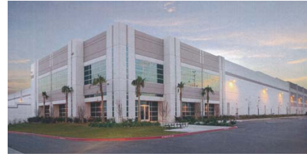
Example of distinguishable front office area
