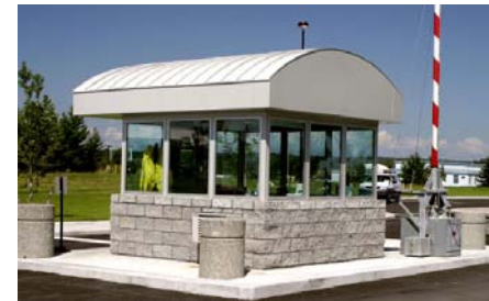
Example of secured entry kiosk
