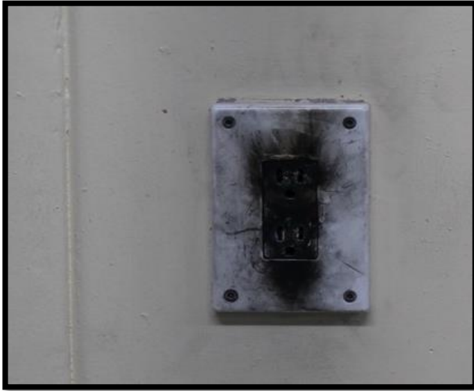
Damaged electrical outlet in housing unit
