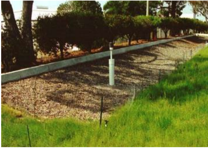
Figure 8-19. Infiltration trench
