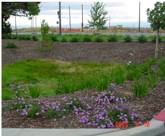
Figure 8-1. Bioretention Area, Fremont
