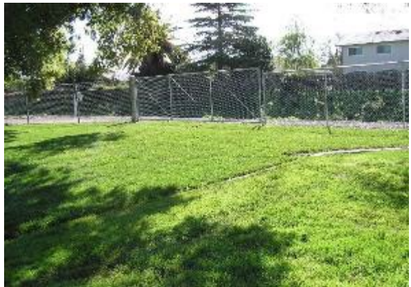
Figure 3-3. Pleasanton Sports Park includes a turf block fire access road.
