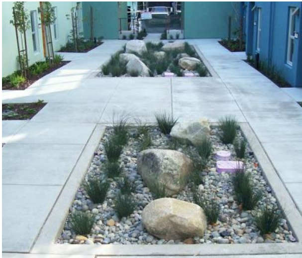
Figure 8-10. At-Grade Flow-Through Planters Source: City of Emeryville
