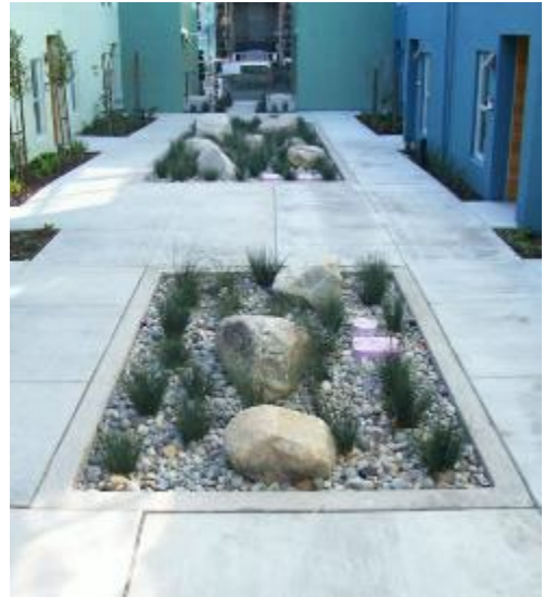
Figure 3-6. Flow-through planters are incorporated into the landscaping in a dense, urban setting in Emeryville.
