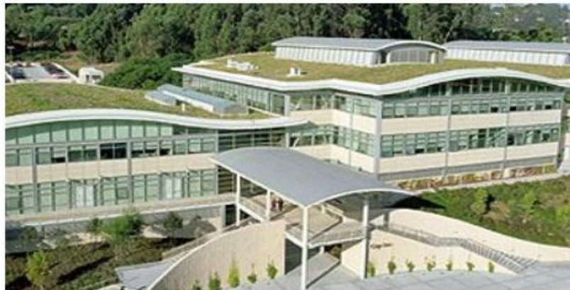
Figure 8-36. Extensive Green Roof at Gap Corporate Headquarters, San Bruno Source: William McDonough & Partners
