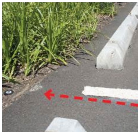
Figure 7-13. Stormwater runoff enters the stormwater facility through the 3-foot space between these wheelstops. The design could be improved by providing more of a drop in grade between the asphalt and landscape area.
