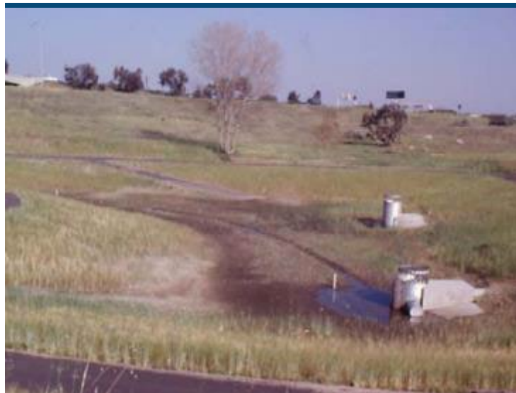
Figure 8-22. Extended detention basin Source: CASQA, 2003
