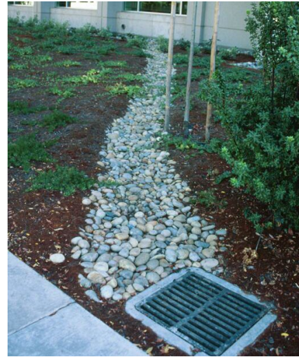
Figure 9-4. Draining roof runoff to a landscaped area is an example of hydrologic source control.
