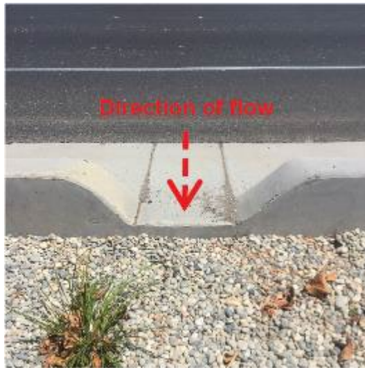
Figure 7-7. Standard Curb Cut.
