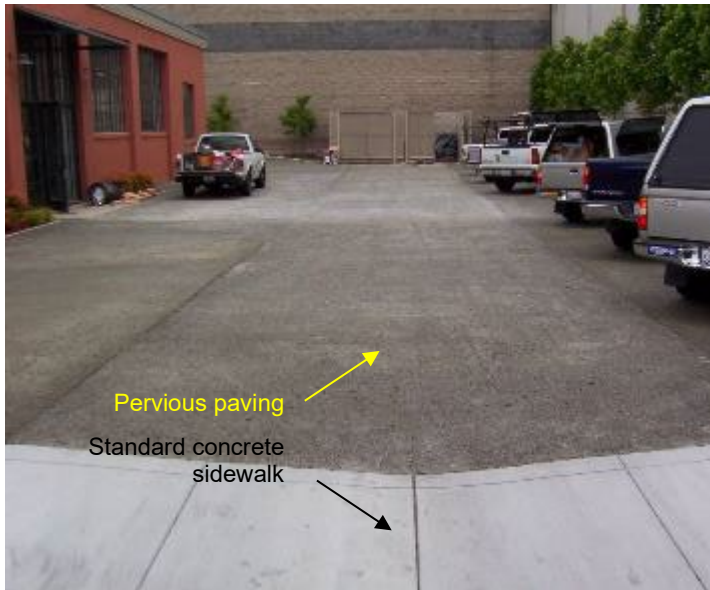
Figure 8-26. Parking Lot with Pervious Concrete Pavement, Emeryville
