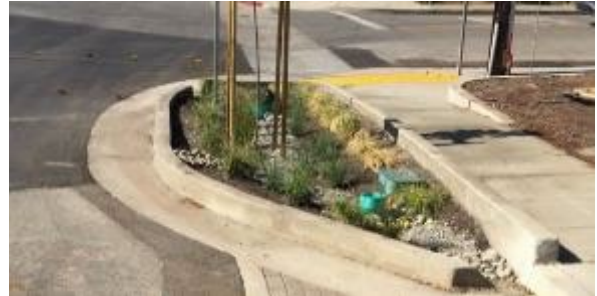
Figure 4-1. Bioretention Curb Extension in Union City
