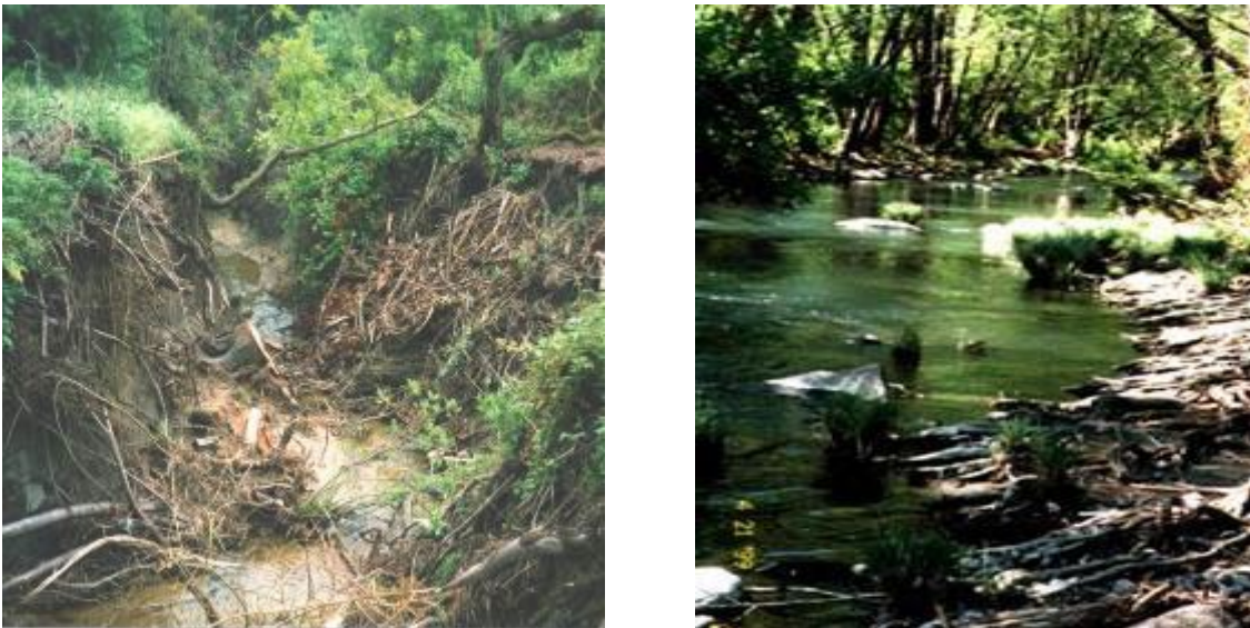
Figure 2-2. Hydromodification impacts on a creek (left) and Creek with natural banks (right).
