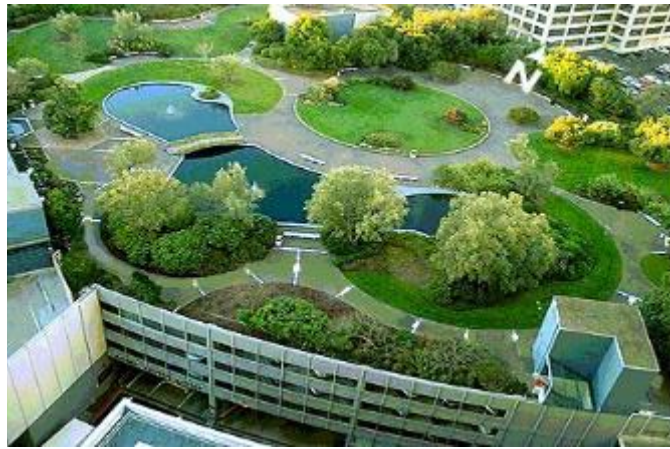
Figure 8-38. Intensive Green Roof at Kaiser Center, Oakland.
