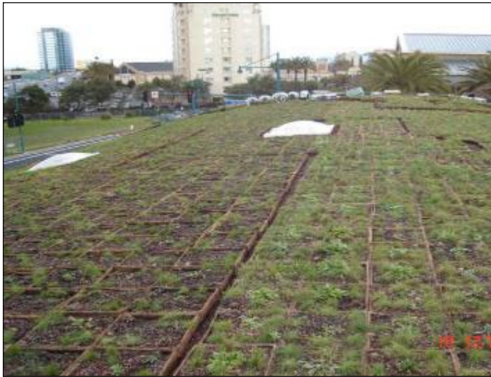
Figure 8-34. Extensive Green Roof in Emeryville
