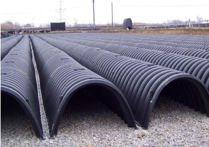
Figure 8-44. Subsurface Retention/Infiltration System Installation Under a Parking Lot
