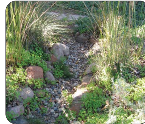
Dry creek infiltrates and conveys runoff.
