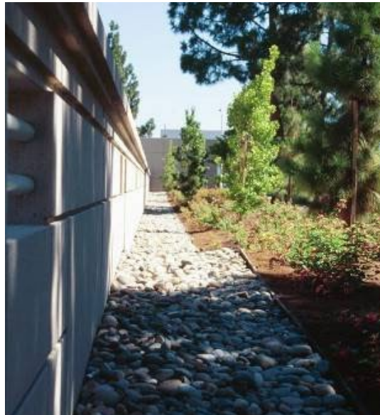
Figure 8-20. Infiltration trench next to parking structure, Palo Alto. Source EOA, Inc.
