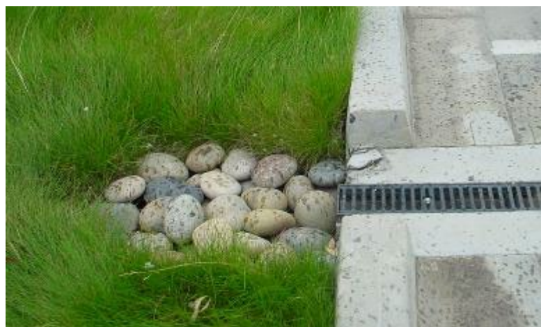
Figure 7-6 Cobbles are placed at the inlet to the stormwater treatment measure to help prevent erosion.
