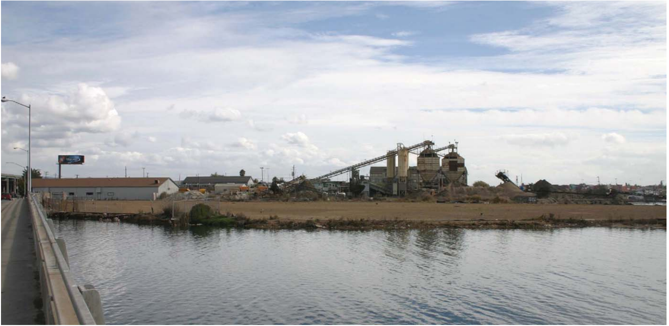
Existing view from Embarcadero at Lake Merritt Channel looking southeast (VP5)
