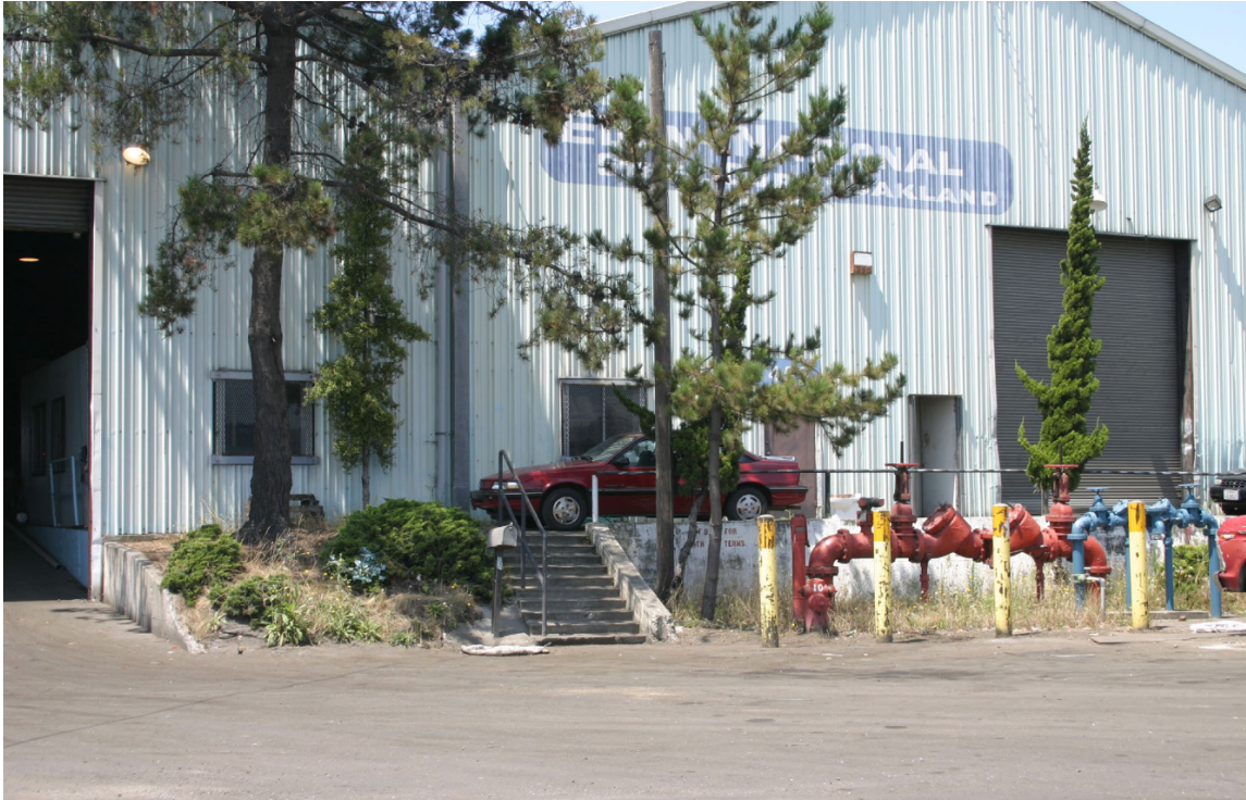
Existing internal view looking southwest (VP13)
