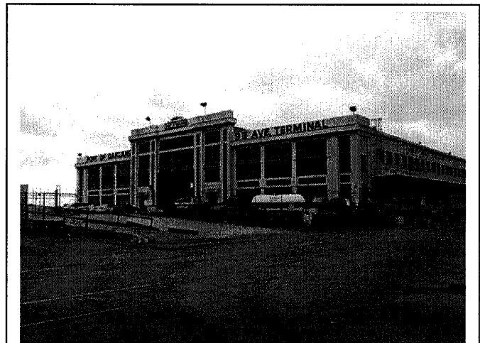
9 th Avenue Terminal (Port of Oakland Bldg #H-309) Carev & Co., October 2004
