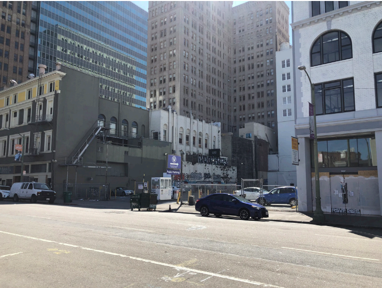
3 - View towards site from east
