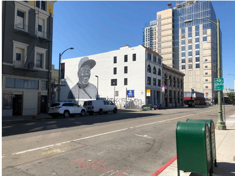
1 - View to site from south
