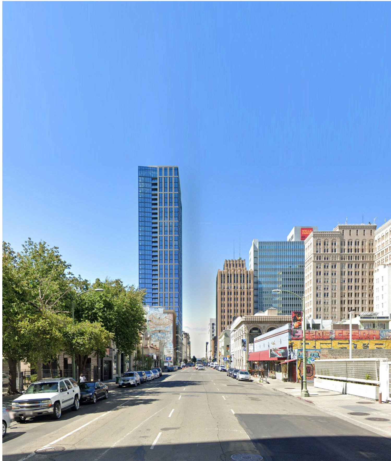
VIEW FROM CITY FRANKLIN LOOKING SOUTH
