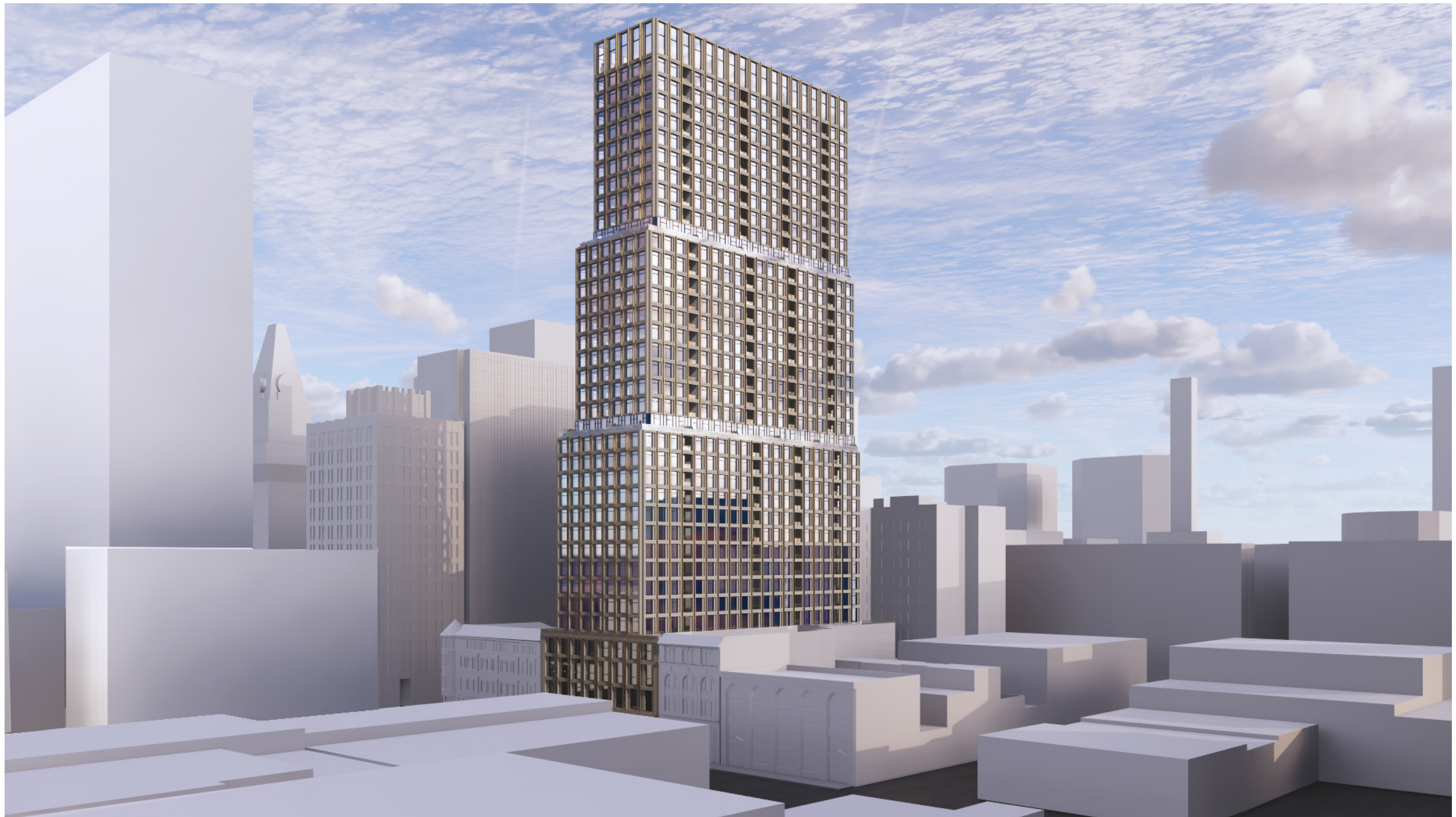
OVERALL LOOKING SOUTH-WEST
