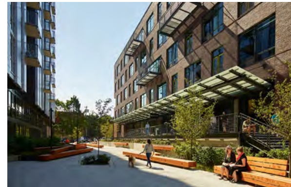
Figure 54: Community Room along Paseo
