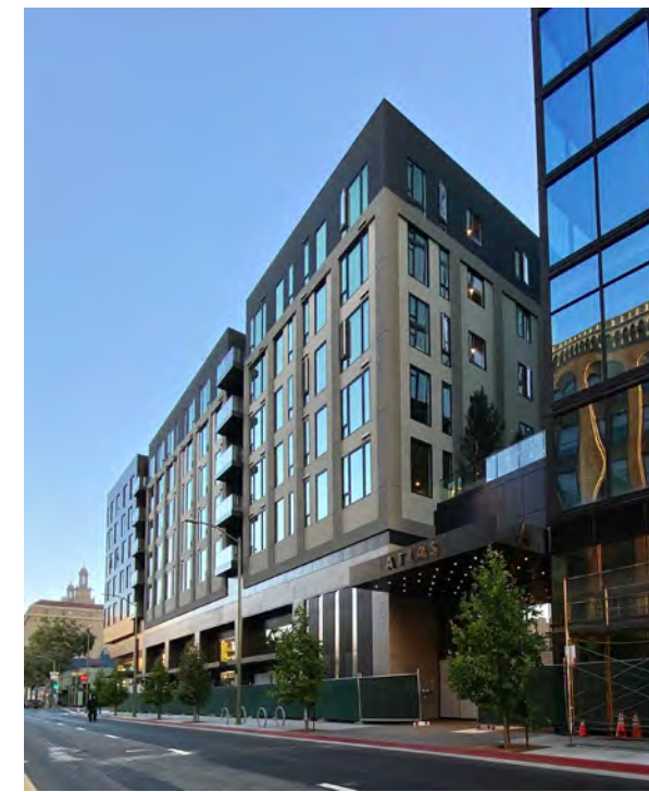
Figure 59: Mass Break between Buildings C and D
