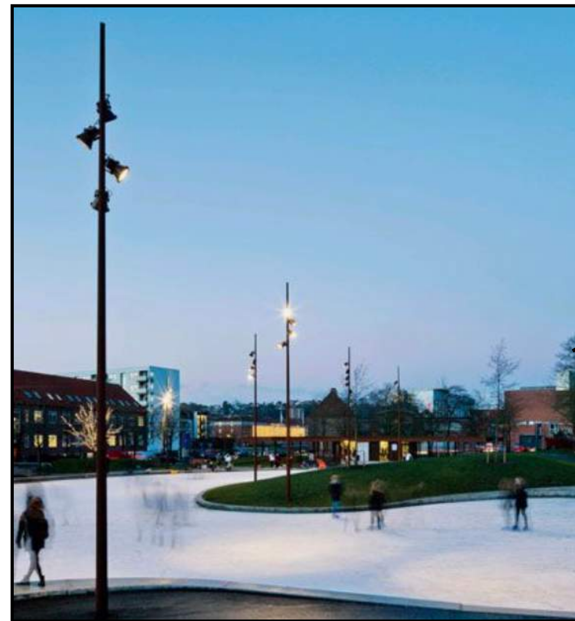
General lighting - Multi-headed pole
