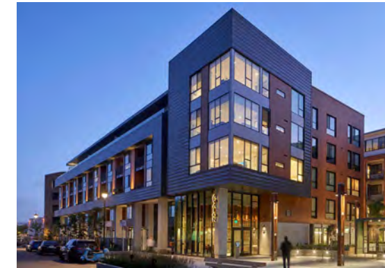
Figure 31: Building Corner at 8th and Fallon Streets
