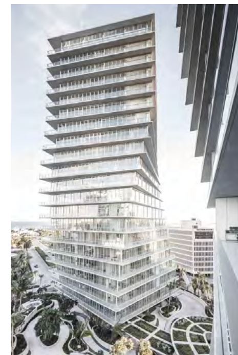
Figure 25: Shaping West Tower Facade
