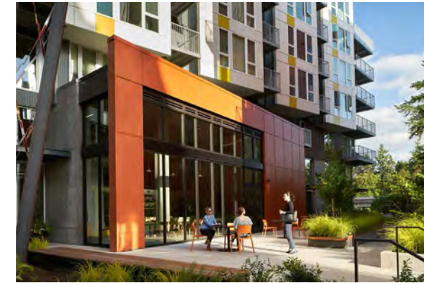
Figure 19: Residential Community Room
