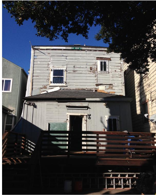
**The siding is warped, and the paint is deeply blighted on the south and east sides. The rear of the house is dilapidated and rotten.**
