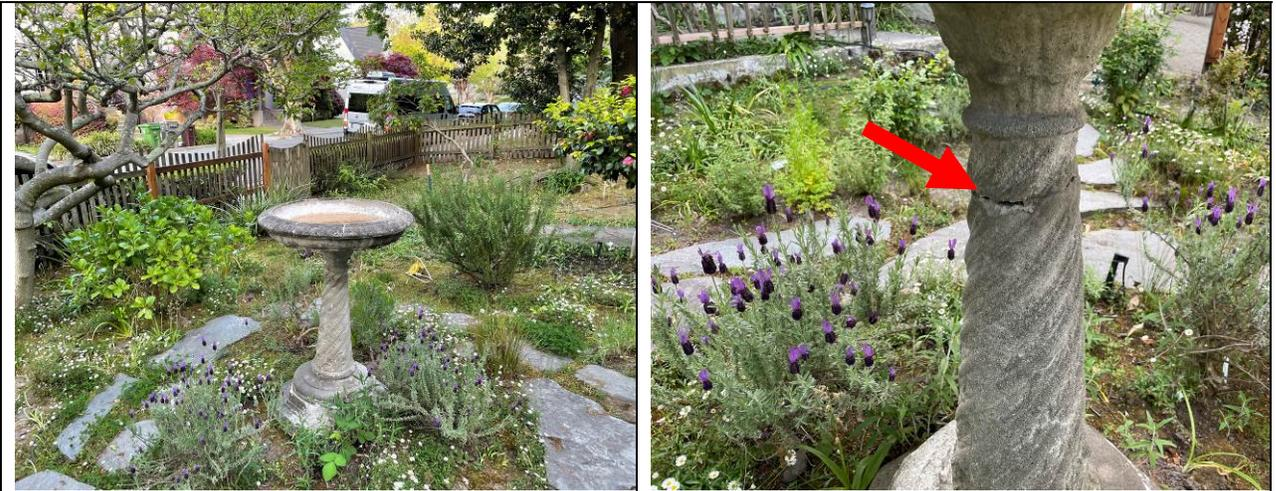
*Work Item #2 - Photo 4 &5 Early if not original bird bath to be repaired. Red arrow is a crack on the pedestal post.*
