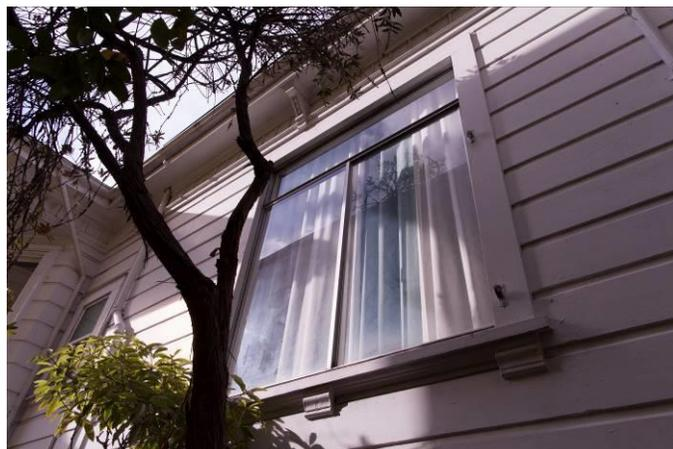
Observe aluminum window frames. Casing appears to be original. Intent is to replace aluminum windows with replica wood windows (double or triple glazed for increase energy efficiency).
