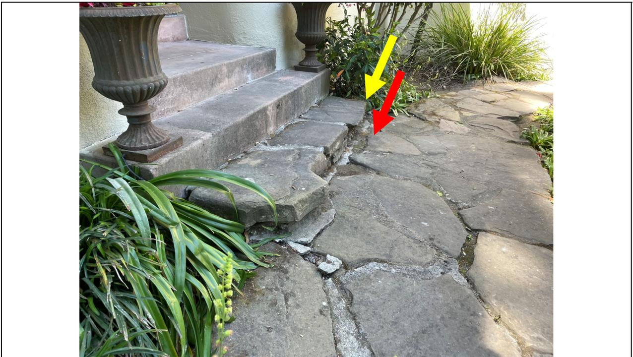
*Work Item #1 - Photo 1 The stone step was installed ~2011 (yellow arrow) and pathway (red arrow) were originally level in 2002. The vertical displacement depicts significant and continued ground settling. Install support foundation under the house.*
