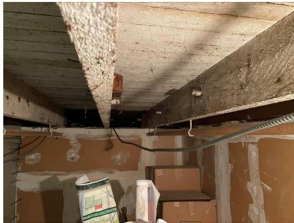
Observe the absence of shear transfer ties or blocking between joists.
