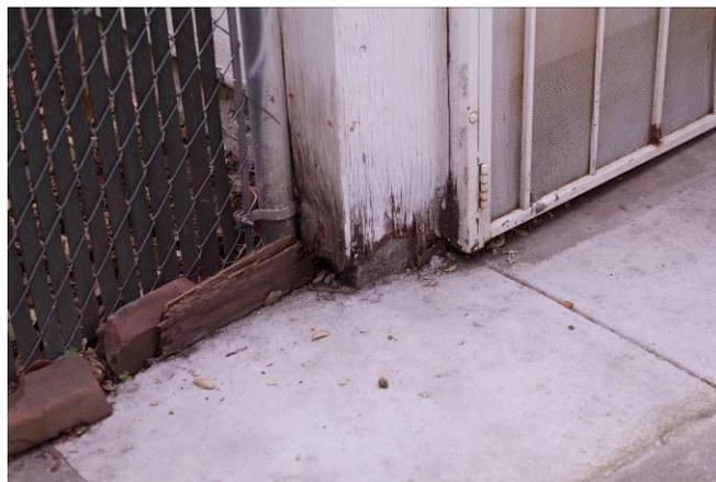
Observe this rotten door casing. All wood with ground contact will be repaired or replaced in kind with historically accurate moldings.
