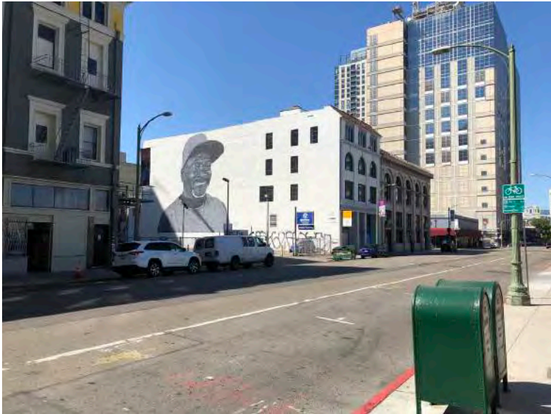
1 - View to site from south
