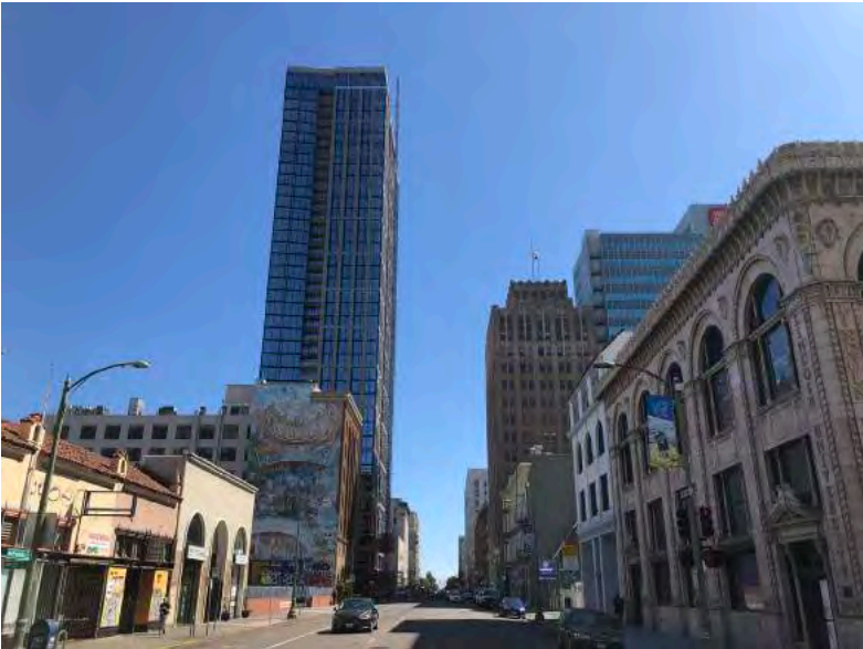
8 - View along franklin ave. to south-west
