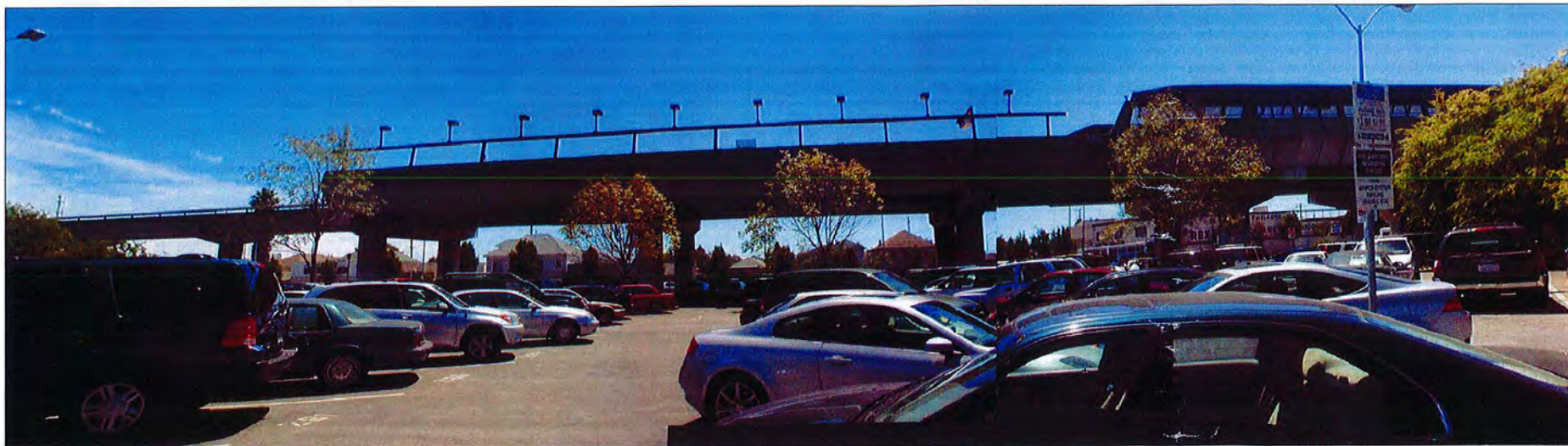
PHOTO #14: FACING SOUTH TOWARDS BART TRACKS
