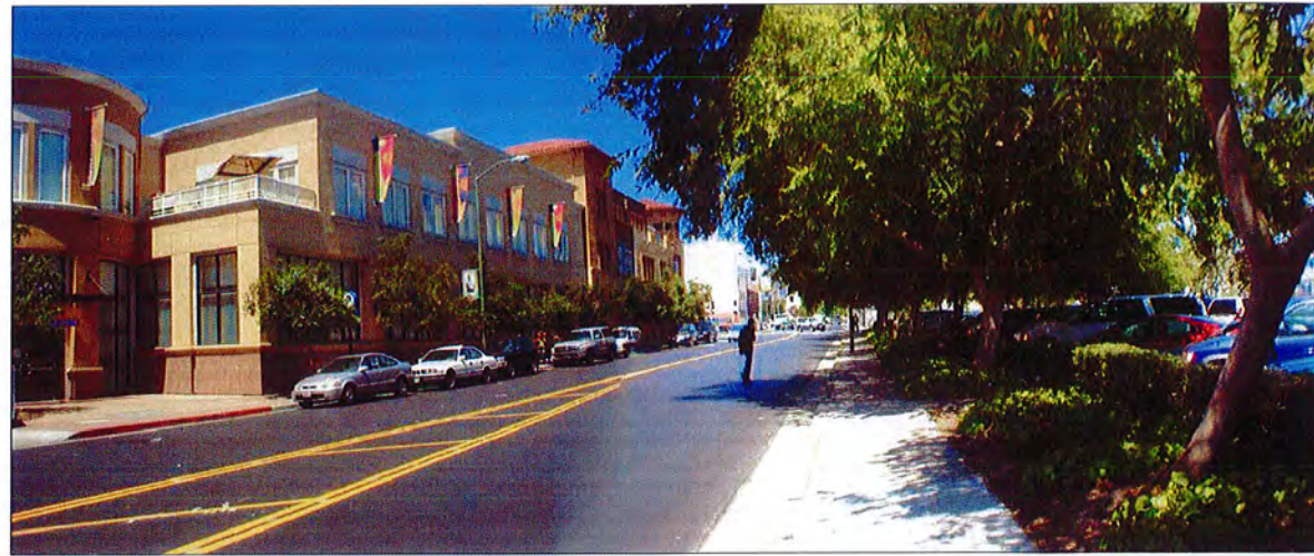
PHOTO #1: FACING NORTH ON 35TH AVENUE (FRUITVALE VILLAGE ON THE LEFT, PROJECT SITE ON THE RIGHT)
