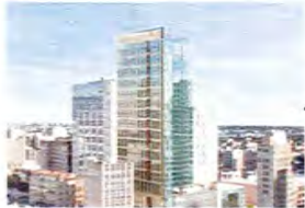
1640 BROADWAY Lennar 380' Under Construction
