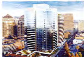
601 CITY CENTER Shorenstein 24 story Under Construction
