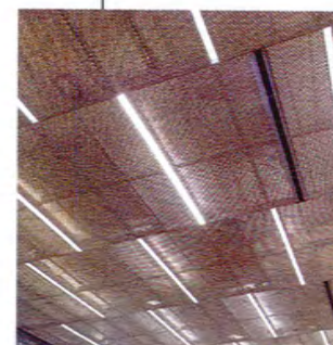
METAL SOFFIT WITH LIGHTS
