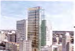
1640 BROADWAY Lennar 380' Under Construction
