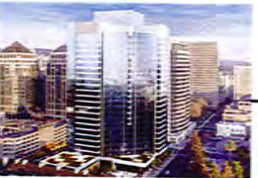
601 CITY CENTER Shorenstein 24 story Under Construction
