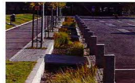
BIORETENTION BASIN w/ METAL GRATE
