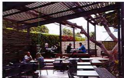
OVERHEAD PERGOLA STRUCTURE
