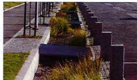
BIORETENTION BASIN w/ METAL GRATE
